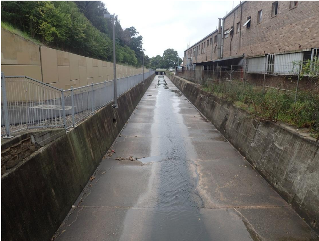
Figure 5 Wolli Creek concrete-lined trapezoidal channel upstream of Kingsgrove Road
