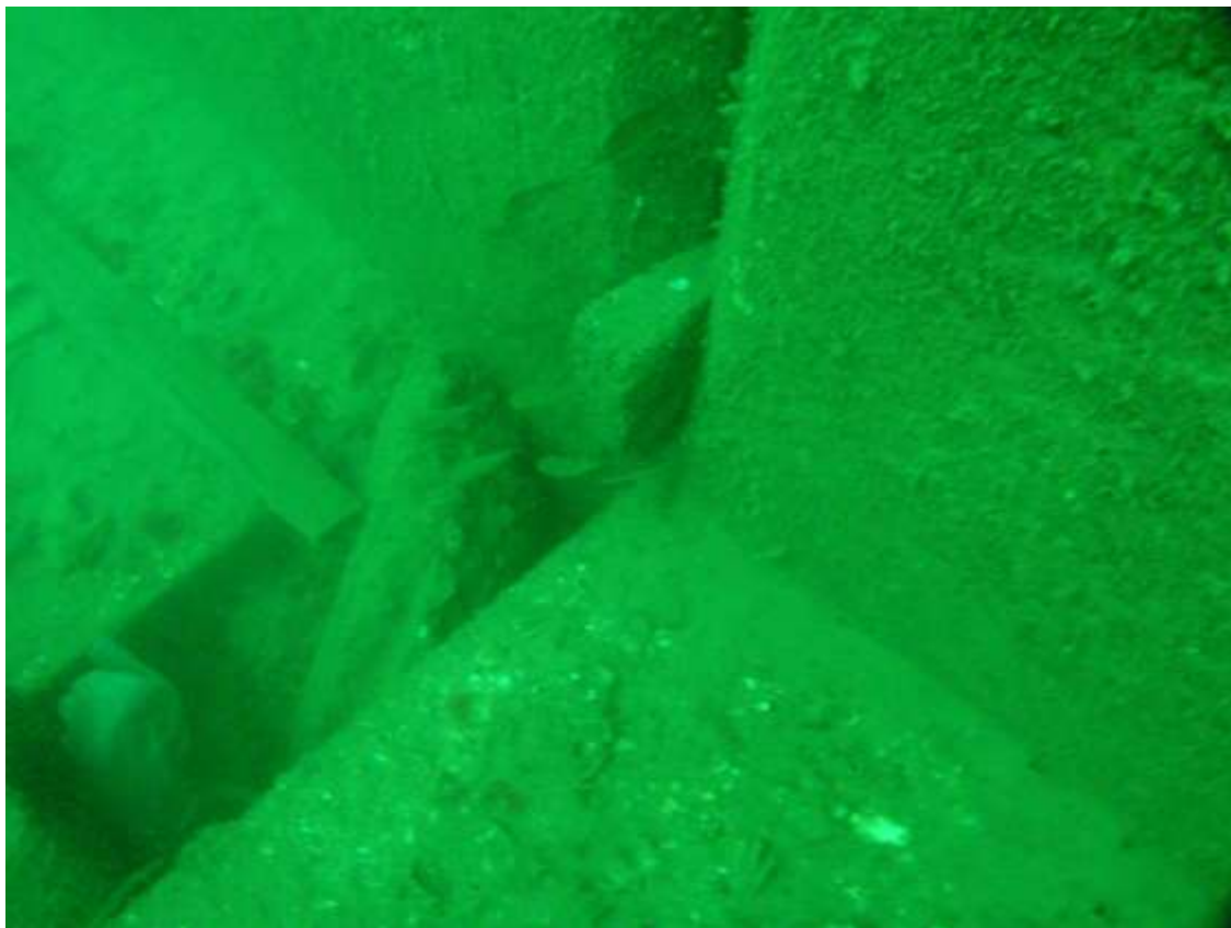
Figure 9 Each caisson has a broad concrete base and there are gaps of about 5 centimetres wide between each caisson unit with rubber gaskets between the units. The exposed portions of these gaps provide shelter habitat for fish, in this case cardinal fish.
