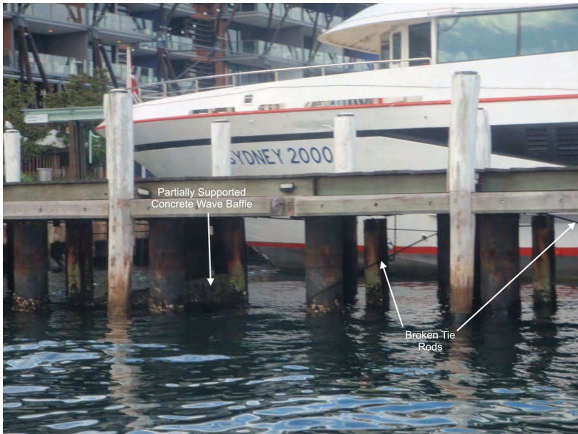
Figure 4 Middle Section of Wharf 10 Jetty showing a partially supported concrete wave baffle and a number of broken tie rods.
