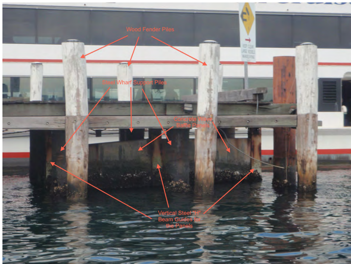
Figure 3 Outer section of Wharf 10 Jetty showing two suspended wave baffles
