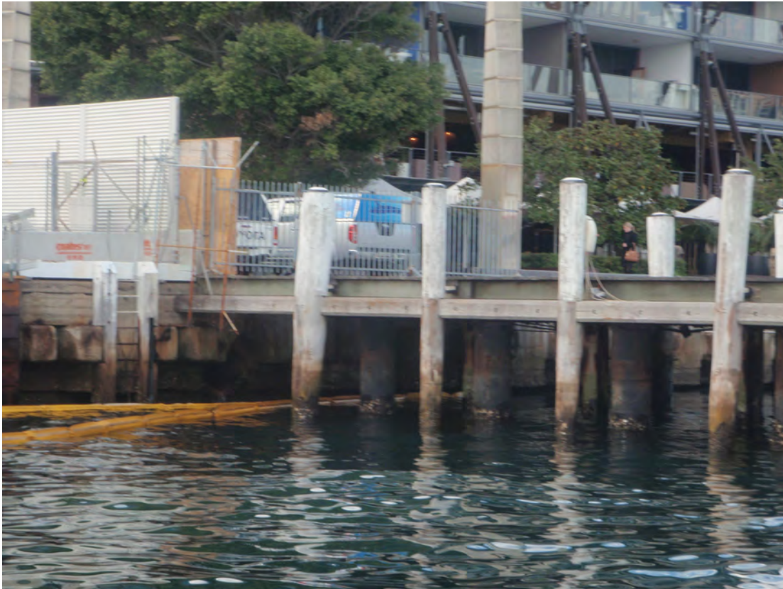
Figure 5 View of sandstone and concrete retaining wall at the shore-end of Wharf 10 Jetty. The floating boom and construction fencing to the left side of the wharf are part of the Barangaroo construction works, and there is a stormwater outfall to the left of the jetty.
