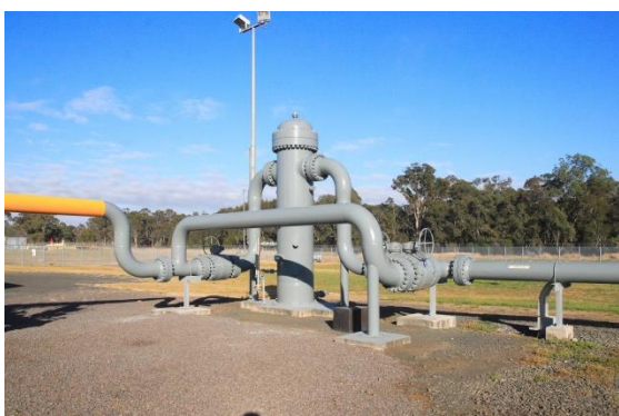
Plate 1-5 Bulk liquid separator and associated pipework
