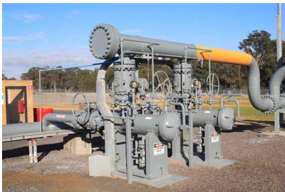
Plate 1-3 Dry gas filters and associated pipework
