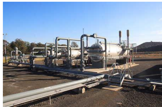
Plate 1-4 Water bath heaters (three) and associated pipework
