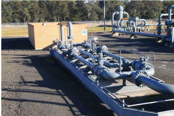
Plate 1-1 Metering equipment (foreground) and regulator for gas delivery to the Central Trunk (inside masonry enclosure)
