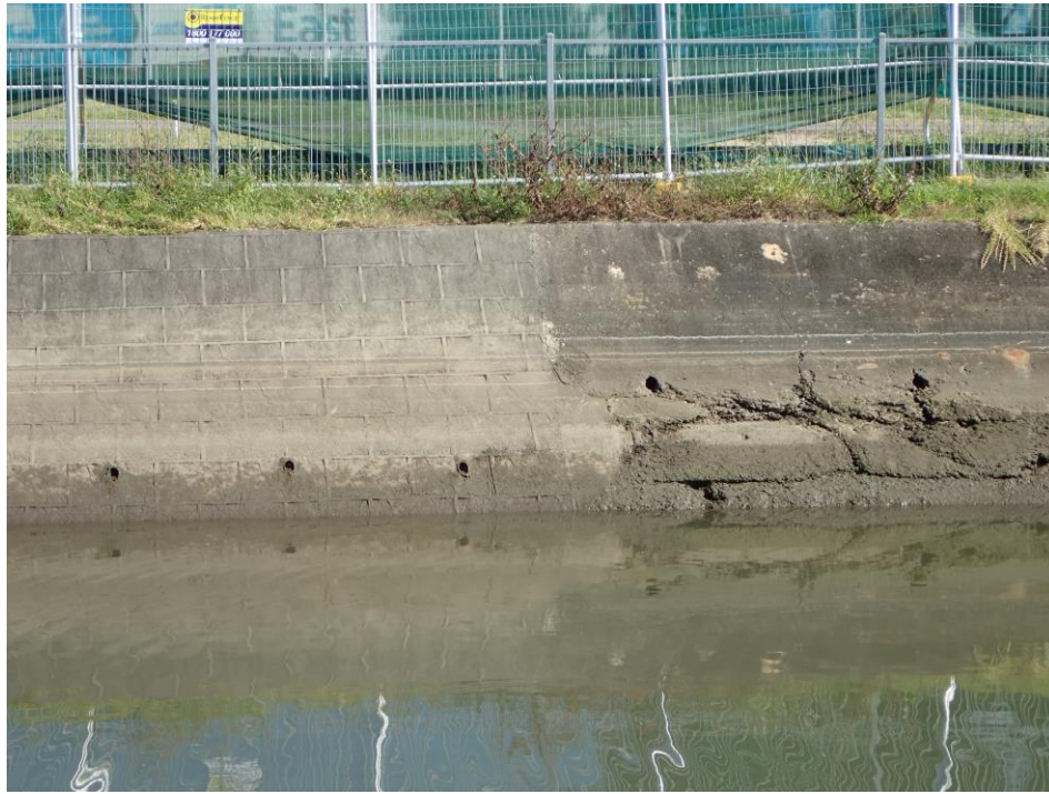
Figure 3.5 Detail of the east bank of the canal showing earlier (right) and later (left) sections of the wall. Stormwater Outlet 2 will pierce a section of canal wall that is likely earlier and in a poor condition.
