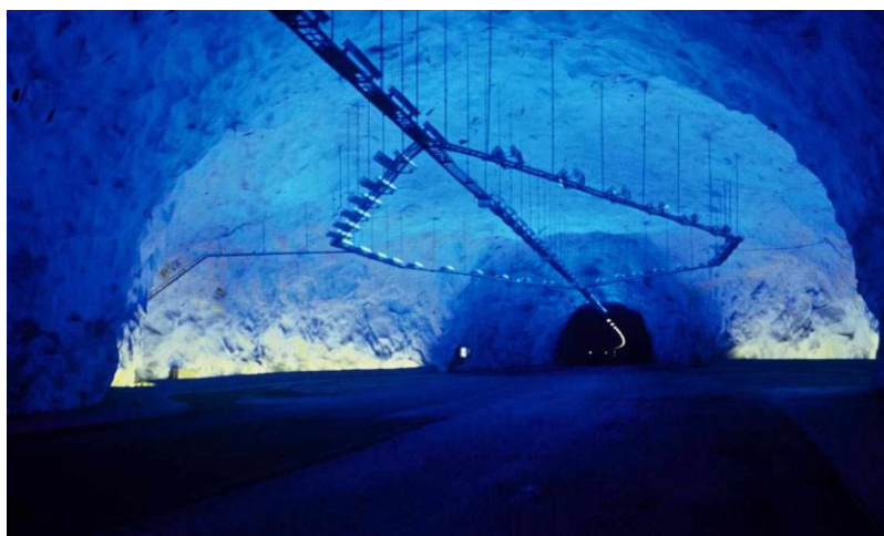
Image 1.6 – Image of the Lærdal Tunnel, Norway
