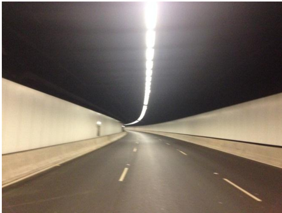
Image 1.4 – Example of traditional tunnel lighting Lane Cove Tunnel, Sydney, Australia xiv
