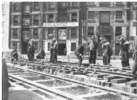
Figure 2.37 Chopping up Road at Circular Quay to lay new tram lines, undated. (Source: Sam Hood Collection 1872-1953, SLNSW)
