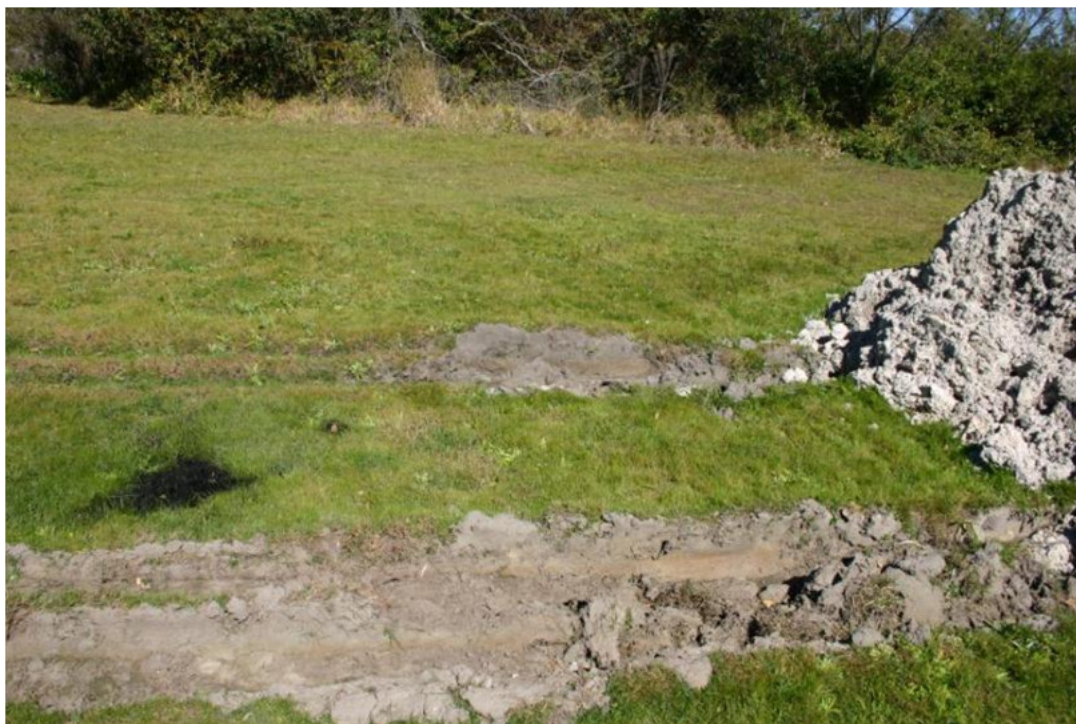
Figure 6.2 Soft silty/sandy fill used to create flat area across majority of Aquatic Drive study area.
