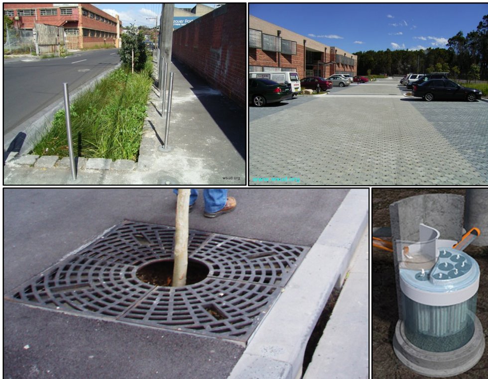
Figure 1 - WSUD techniques [Clockwise from top left: raingarden scheme in Cremone Street, Melbourne (wsud.org 2012), permeable pavement in a Sutherland car park (wsud.org, 2012), Humes JellyFish, tree pit (Auckland Council 2012)]
