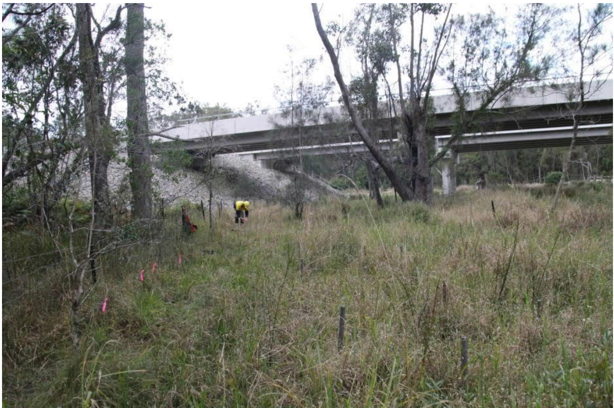
Plate 33: Hairy Joint Grass receival site at Mitchell Rd, looking east. HJG plants within 2m of the fence had died back 2-3 months ago but the dead stems were still visible. July 2019
