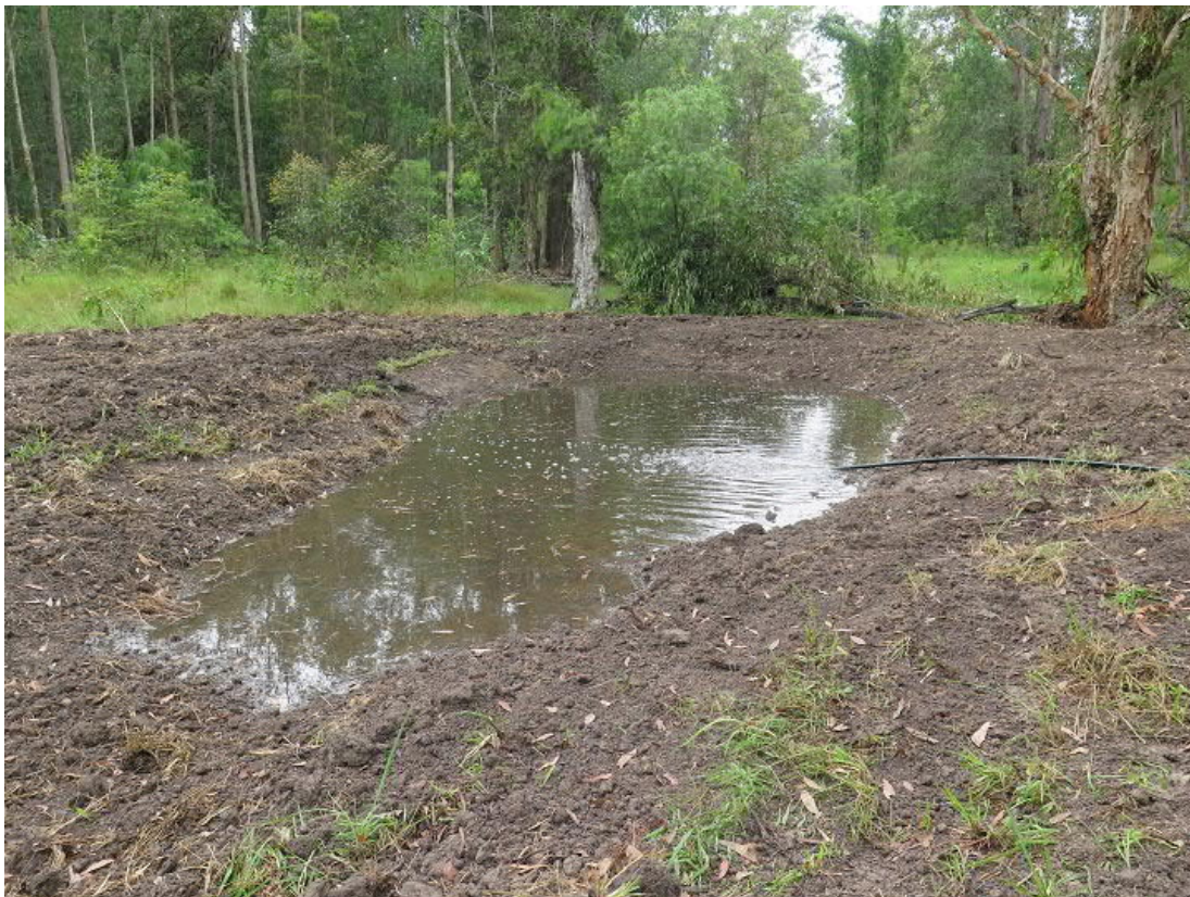
Plate 36: Filling one of the excavated Rotala ponds near Tabbimoble Ck, November 2017
