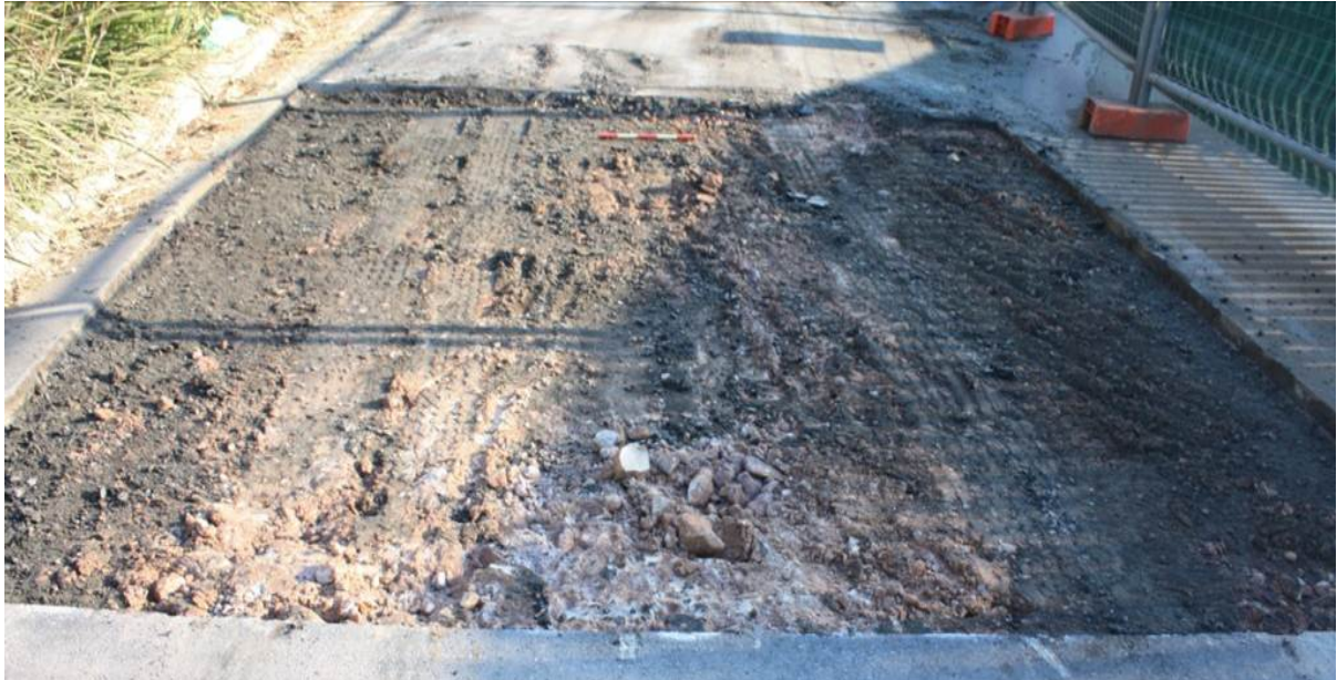
Plate 3: Test Trench 1, view north showing road surface, road base [050, 051], gutter and kerb [052, 073]; scale 500 millimetres
