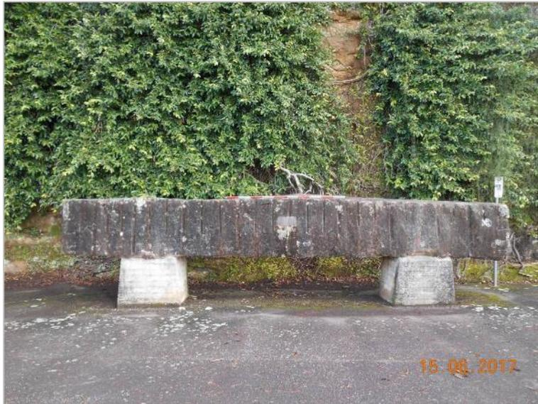
**Plate 16: An example block of cyclopean masonry located next to Cordeaux Dam wall (Niche 2017)**
