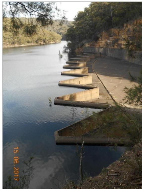
**Plate 30: The redesigned sawtooth/labyrinth spillway weir (Niche 2017)**
