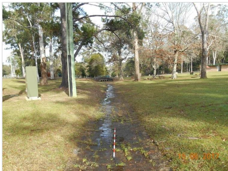
**Plate 5: An original broad stone flagged drain which is still in use (Niche 2017)**
