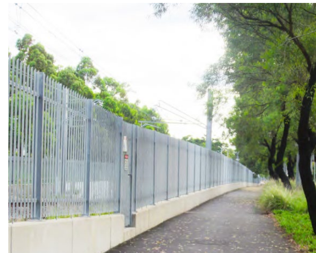
Homebush, Sydney. Rail corridor security fences should be robust, easily maintained, modular systems that are readily integrated with other urban design elements such as retaining walls. (Source: AECOM)
