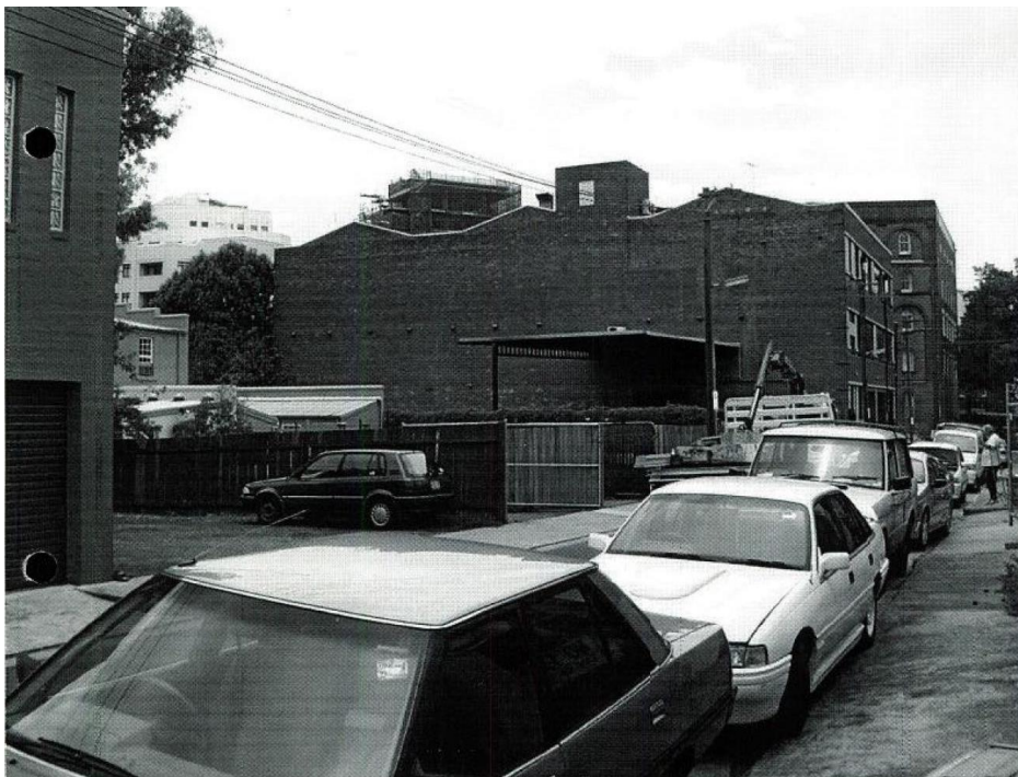
Figure 56: 1999 – Looking southeast from Paternoster Row towards the north elevation of the former Gilbey's Building, with the awning over the loading dock visible at centre. (Source: City of Sydney Archives, D1999/00812, ‘Development Applications/26-32/Pyrmont Bridge
