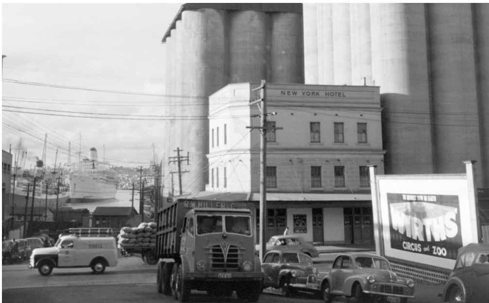
Figure 101: March 1954 – Photograph of the Pyrmont Power Station, by Max Dupain, showing part of the hoarding at the corner of Union and Edward Streets (Source: SLNSW, FL19484880, https://collection.sl.nsw.gov.au/record/nvgPBWJ1 )
