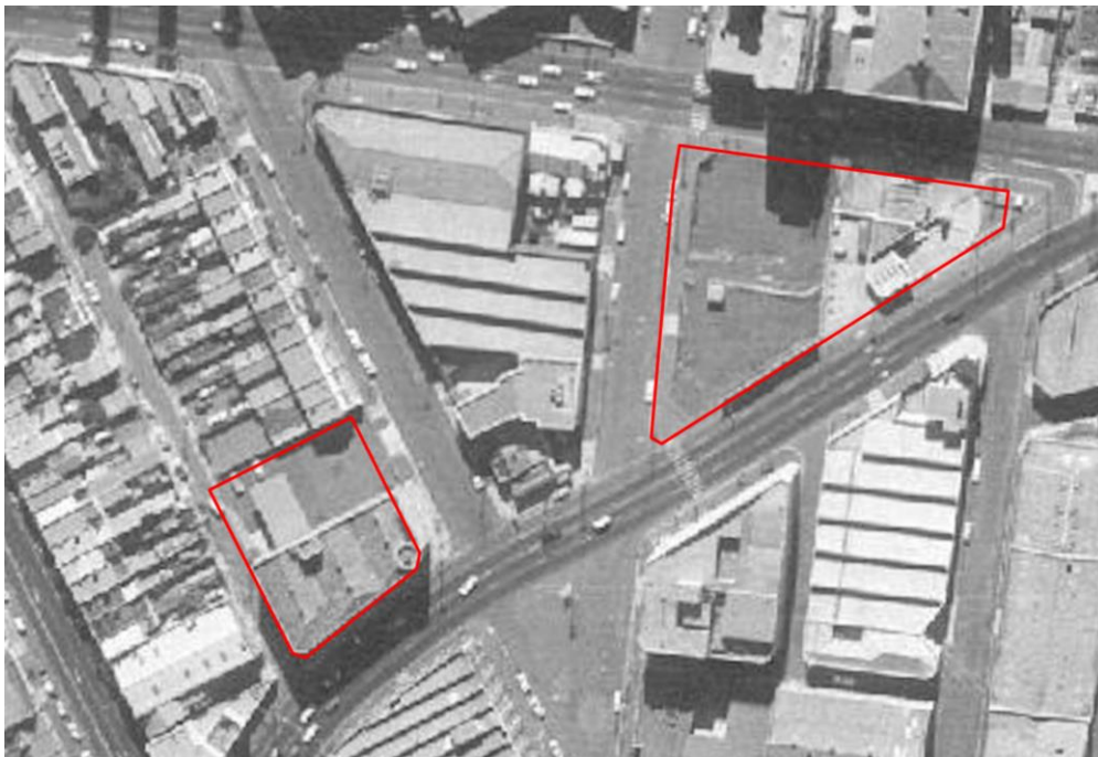
Figure 43: 15 December 1949 – Aerial photograph showing the building under construction (Source: City of Sydney Archives, A-00879983, City of Sydney Aerial Photographic Survey 1949: Image 38)
