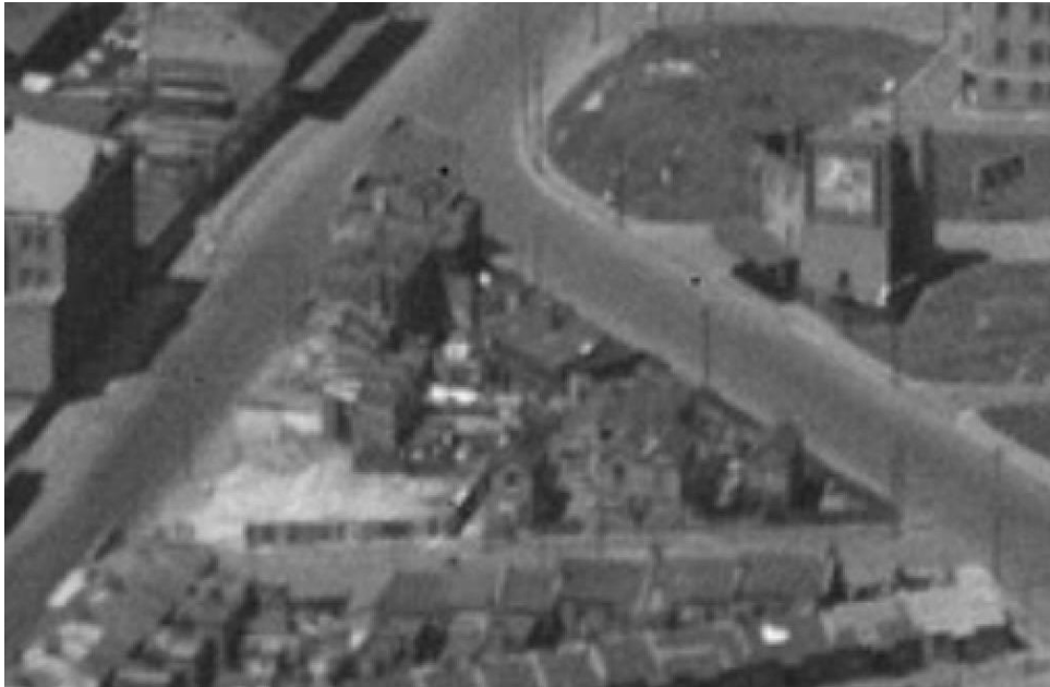
Figure 85: 1930 – Aerial view by Milton Kent, showing the site after demolition of the buildings on the corner of Union and Edward Streets. The image is said to have been taken in 1932, however, by then all the buildings had been demolished (Source: SLNSW, Milton Kent aerial views of Sydney, 1932, FL8812121, https://archival.sl.nsw.gov.au/Details/archive/110367483 )
