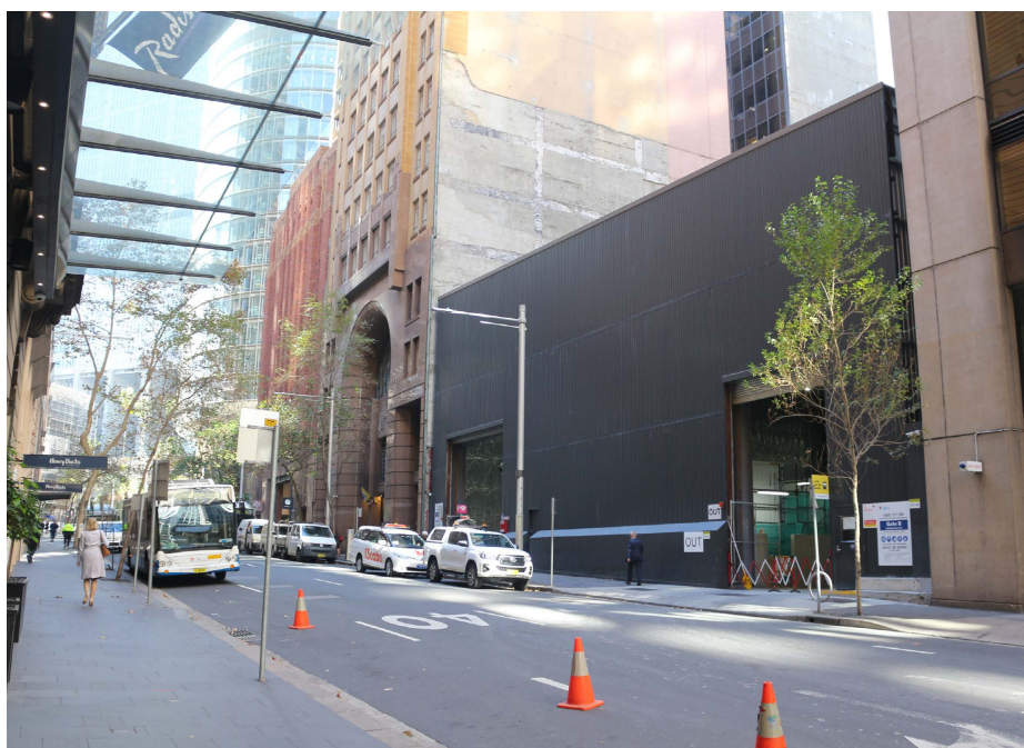
EXISTING ACOUSTIC SHED, BLIGH STREET CONSTRUCTION SITE
