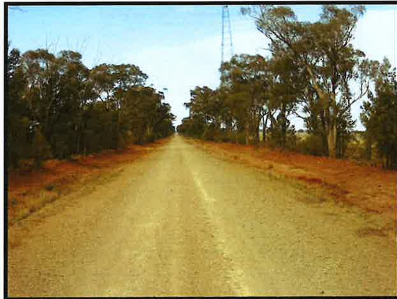
Figure 5 – Crown Camp Road showing 9500-1100 of Crown Camp Road is 8m wide gravel surface road (LSC - July 2021)
