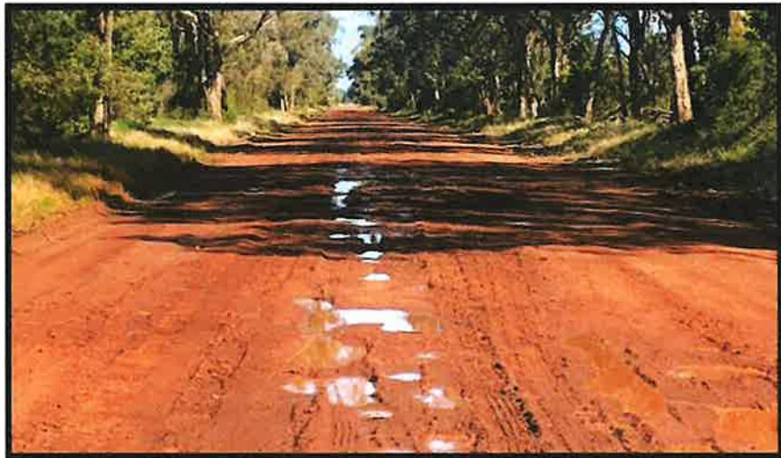
Figure 3 – Crown Camp Road showing 4000 – 9500 of Crown Camp Road is 8m wide gravel/natural surface road (LSC - July 2021)
