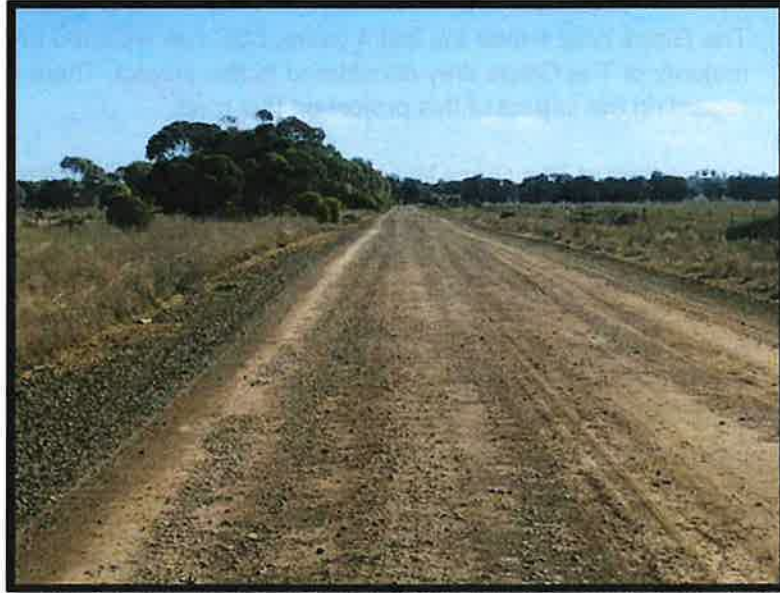
Figure 2 – Crown Camp Road looking west showing 500 – 4000 of Crown Camp Road is 8m wide gravel road (LSC - July 2021)
