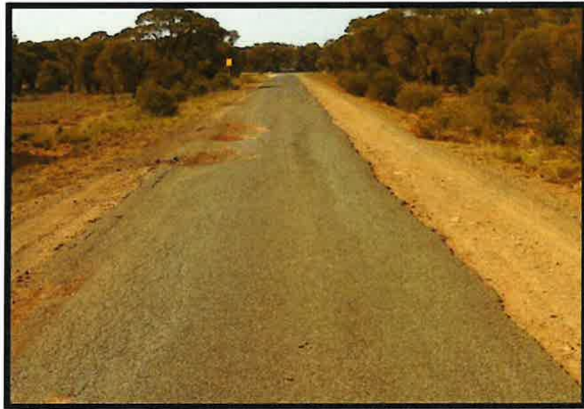
Figure 1 – Crown Camp Road looking east showing seal 3.5m wide for the first 500m, with 3m gravel shoulders (LSC - July 2021).
