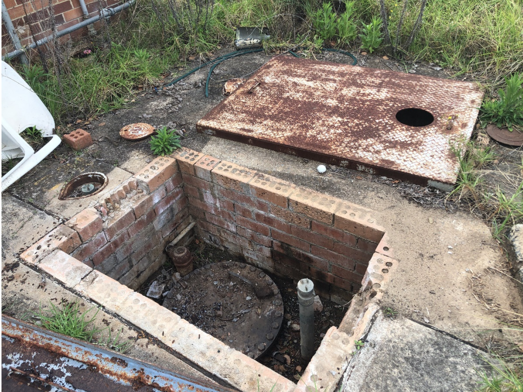
Plate 3 OTC compound diesel UST
