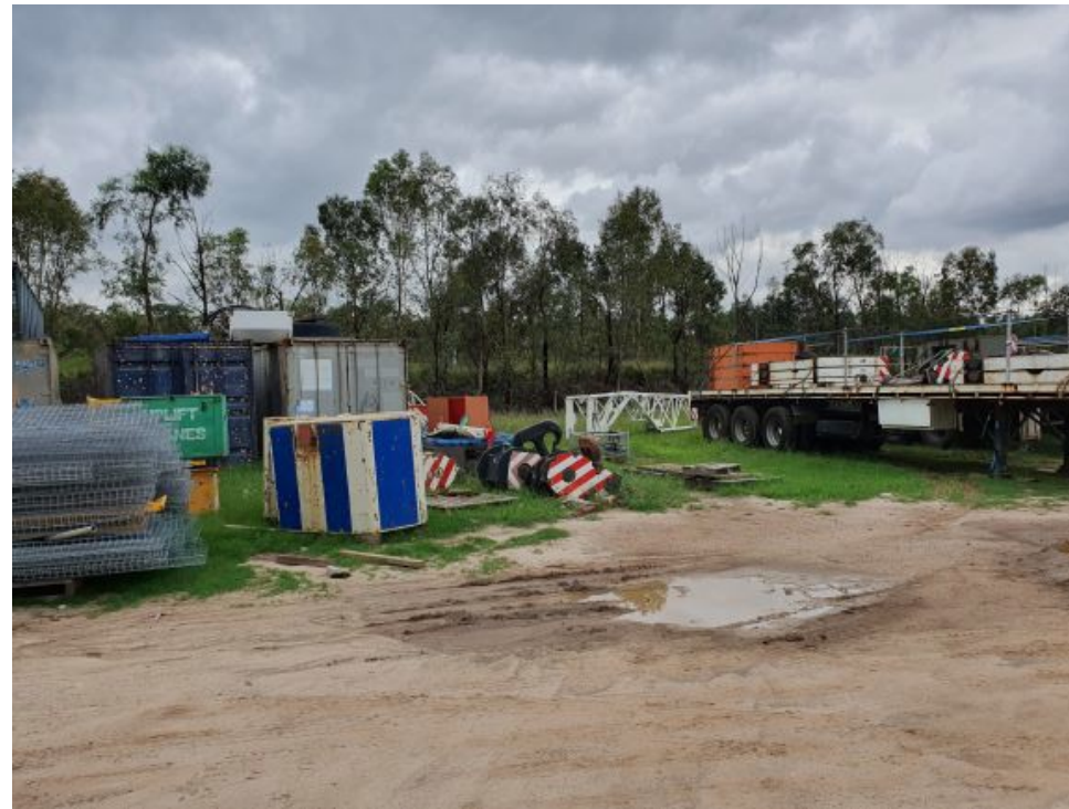
Photograph 29– Area 4: Carpark D – Coates Hire storage area trailers, storage, and construction materials (facing south)
