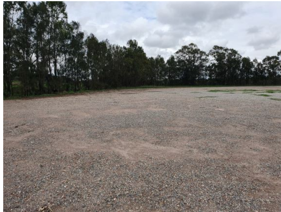
Photograph 20 – Area 3: Carpark C - ground cover (facing west)
