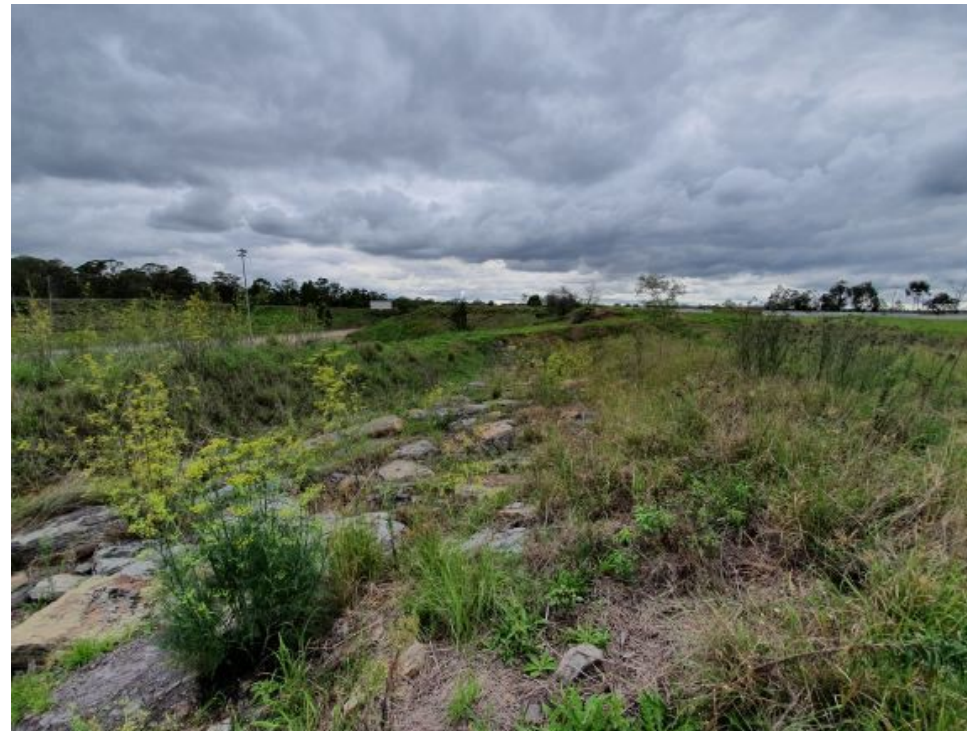
Photograph 35– Area 5: Speedway eastern embankment – stormwater drain (facing south)
