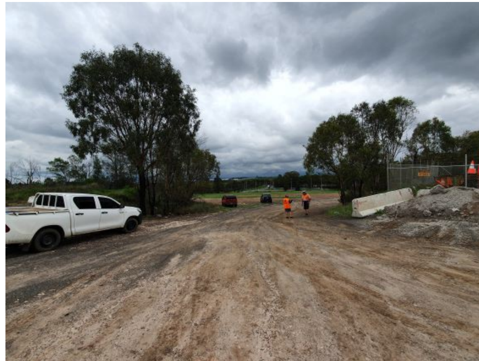
Photograph 23 – Area 4: Carpark D – ground cover (facing south)
