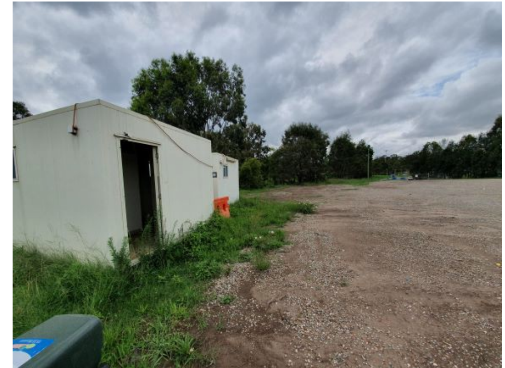
Photograph 18 – Area 3: Carpark C – portable toilets and ground cover (facing east)
