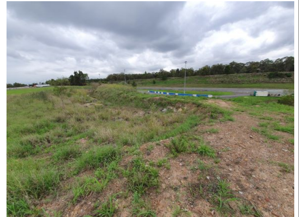
Photograph 36 – Area 5: Speedway eastern embankment – ground cover and stormwater drain (facing north-east)
