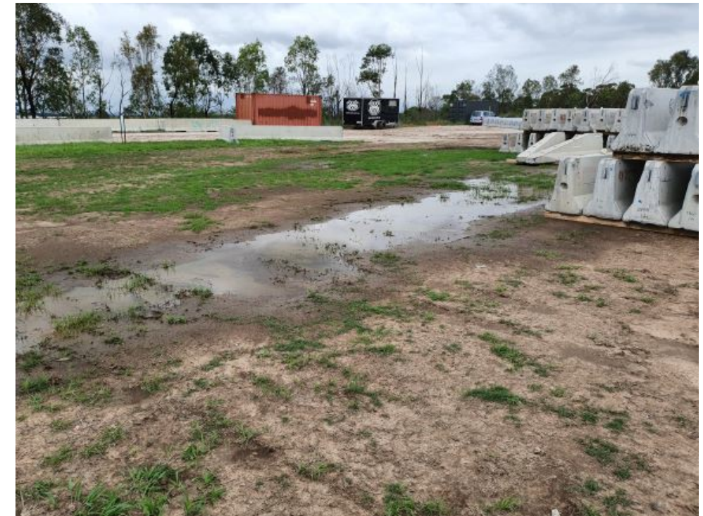
Photograph 30– Area 4/5: Carpark D / Speedway – ground cover and storage containers (facing north-west)
