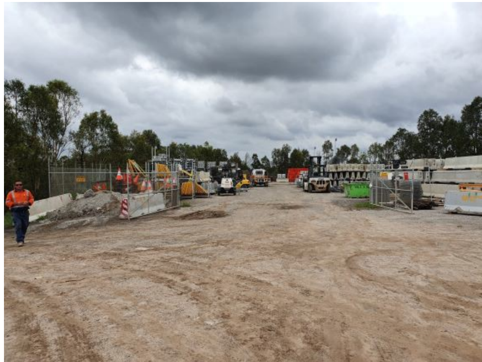
Photograph 22 – Area 4: Carpark D – Coates Hire storage area (facing north)
