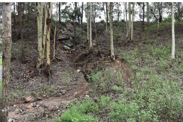
Figure 44 View east of erosional slip on edge of artificial embankment, showing internal fill materials.
