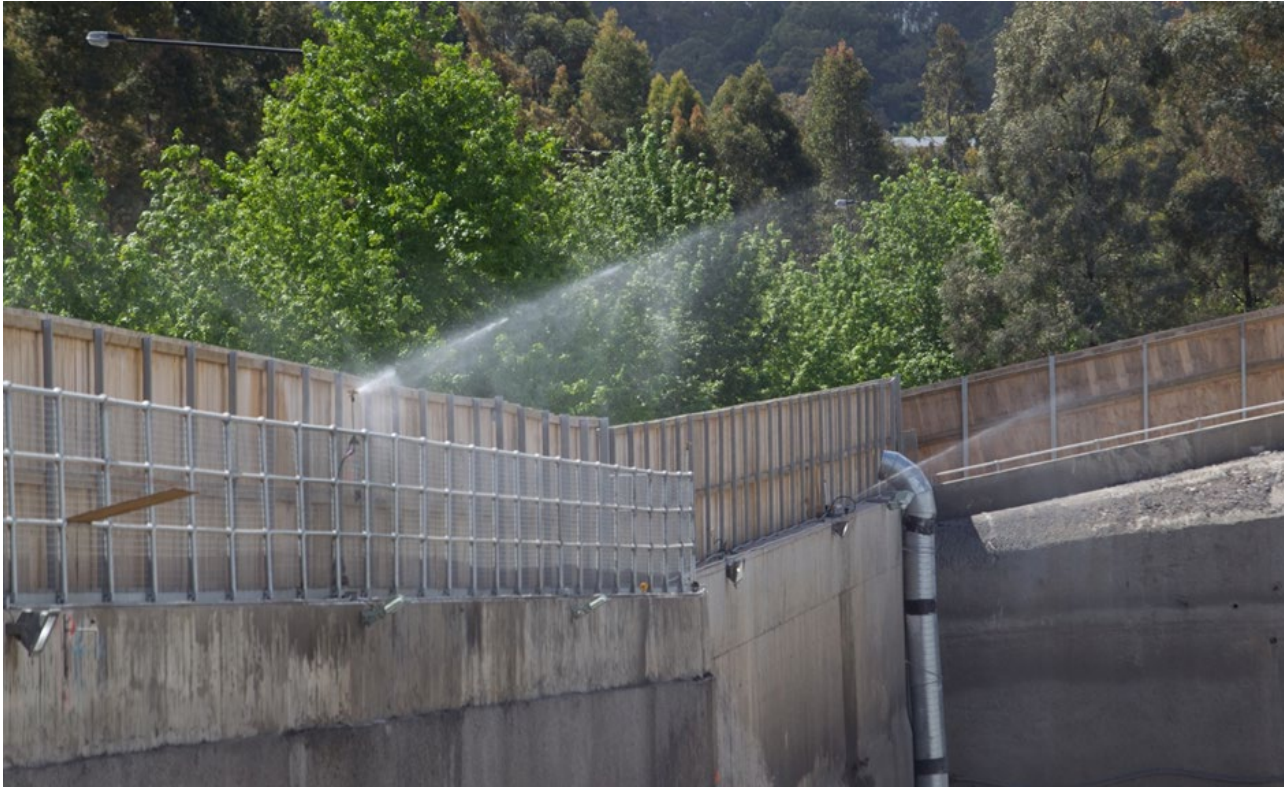
Figure 8 Dust Mitigation at Northwest Station Site
