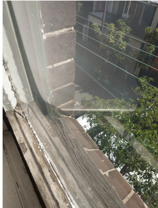
Figure 15 Window framing on northern side of second floor of 125-127 Little Eveleigh Street showing consistent sill and frame without cracks or crevices
