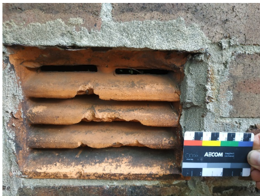
Figure 6 Airbrick at basement level of southern side of 125-127 Little Eveleigh Street
