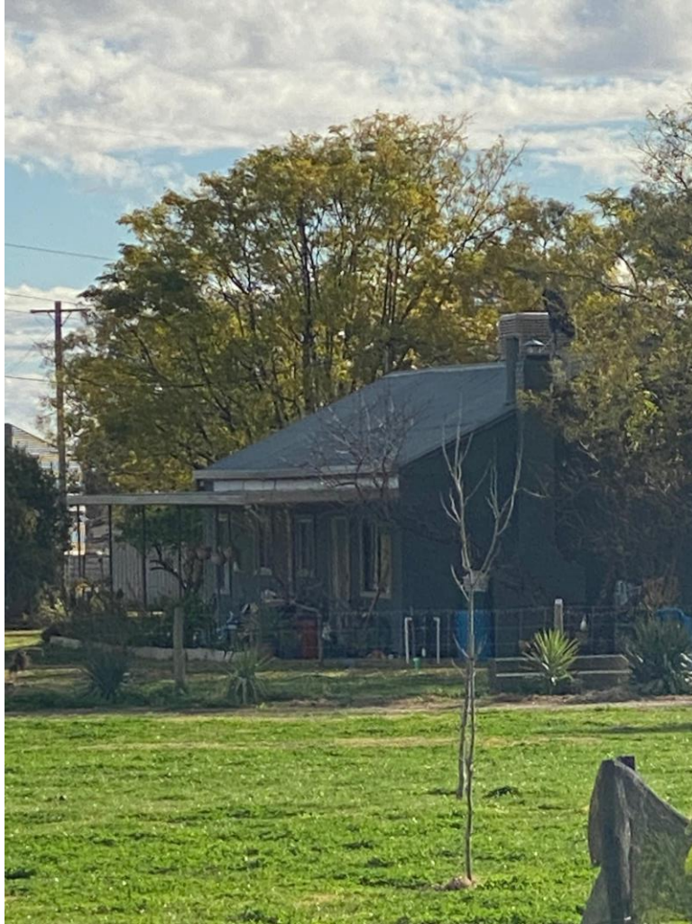
Figure A.2 Photo of R1489 (metal clad Managers Dwelling, corrugated tin roof, single pane windows)
