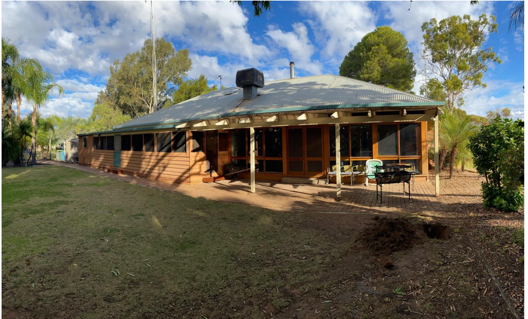
Figure A.3 Photo of R2023 (weatherboard house, corrugated tin roof, single pane windows)
