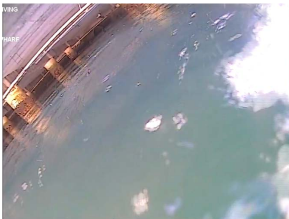
Figure 56: Start of T2, note stormwater drain at end of bay. (Image from T2 (a) Cockle Bay 210705, 00:04).
