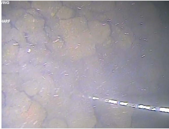
Figure 75: Example of rock batter beginning just to the west of 'C' pile. (Image from T5 (a) Cockle Bay 210705, 03:01).
