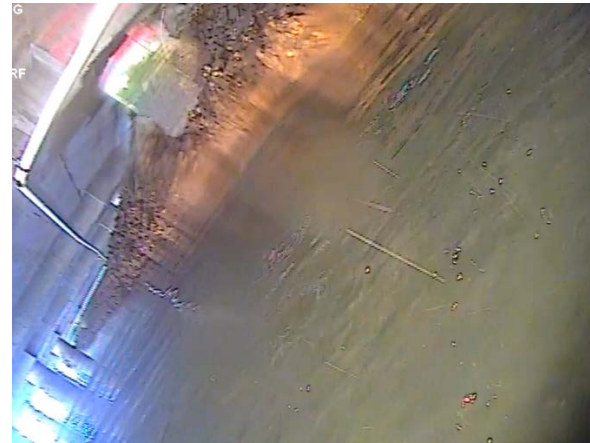
Figure 78: Northern 'D' pile is behind the sheet pile wall. (Image T5 Cockle Bay 210705; 04:59).
