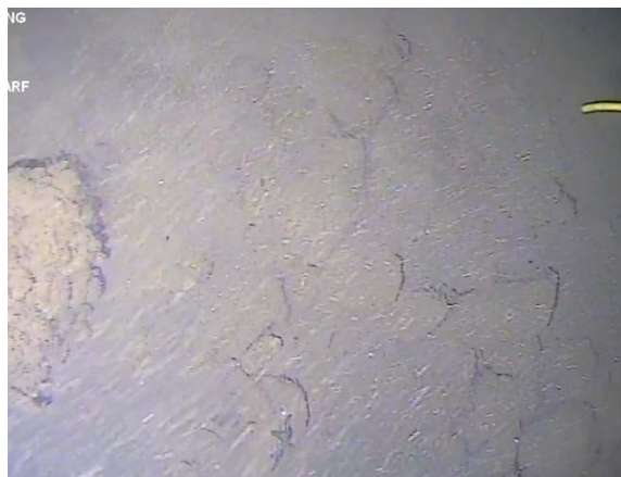
Figure 71: Increase in sediment build-up on the rock batter likely due to stormwater outflow. (Image from T4 (a) Cockle Bay 210705, 05:03).
