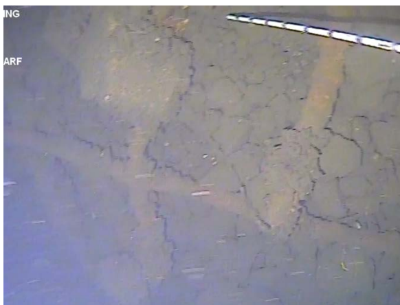
Figure 84: Near the sheet piling there was a number of loose ferrous pipes lying on top of the rock batter. (Image from T6 (a) Cockle Bay 210705; 05:57).
