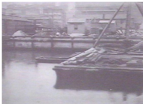
Figure 42 : Completed Monier plate facing of seawall between Wharves 35 and 36, Darling Harbour, 1919. 45
