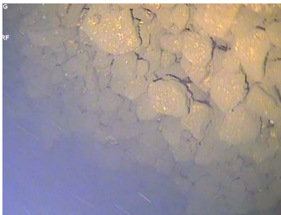
Figure 79: Example of rock batter near the 'C' pile on the northern side of the bent. (Image from T5 (a) Cockle Bay 210705; 05:35).
