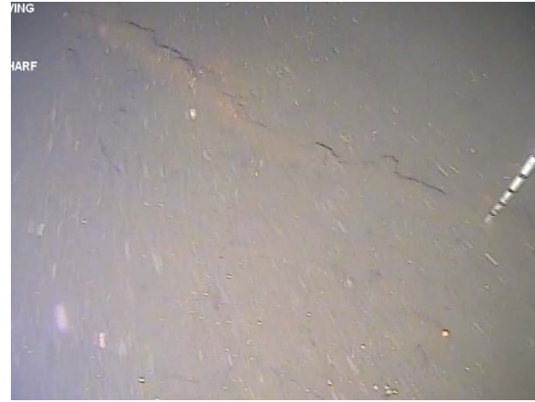
Figure 76: Where the rock batter flattens out, the seabed becomes siltier and there is scattered ferrous piping. (Image from T5 (a) Cockle Bay 210705, 03:40).
