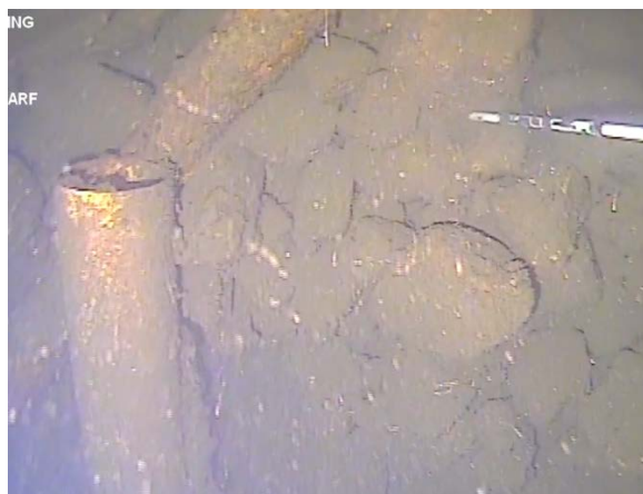
Figure 83: Section of PVC pipe with section of ferrous pipe underneath in the centre of the bent. (Image from T6 (a) Cockle Bay 210705; 04:20).
