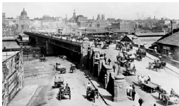
Figure 15: Pyrmont Bridge, facing east, 1907. 22
