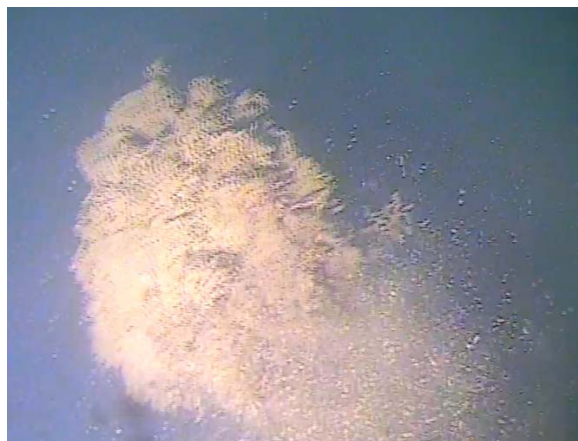
Figure 81: Degraded timber, 500 mm high and 120 mm diameter. (Image from T6 (a) Cockle Bay 210705; 00:43).
