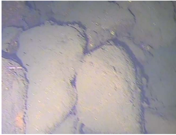
Figure 92: Example of rock batter at southern 'B' pile. (Image from T8 (a) Cockle Bay 210705; 03:44).
