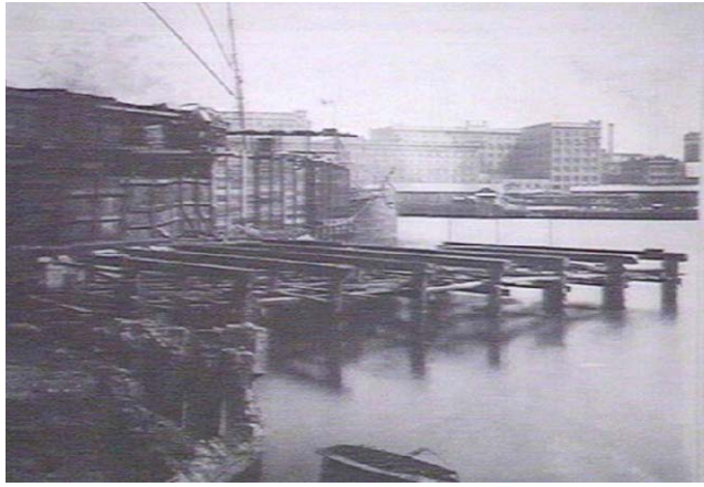
Figure 43 : Construction of Wharf 36, Darling Harbour, 1918, showing what appears to be a Monier plate faced seawall at the base of the wharf, fronting the northern edge of the Jones Bros. Wharf. 46
