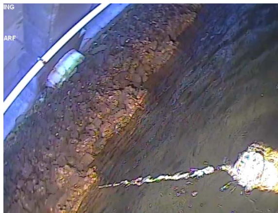
Figure 87: Sheet pile wall at eastern end of transect holding up rock batter. (Image from T7 (b) Cockle Bay 210705; 02:17).
