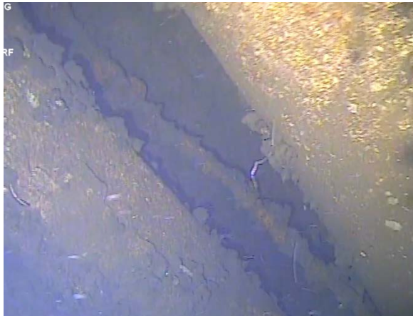
Figure 77: The southern 'D' pile (right of image) is 300 mm to the west of the sheet pile wall. (Image from T5 Cockle Bay 210507, 04:08).
