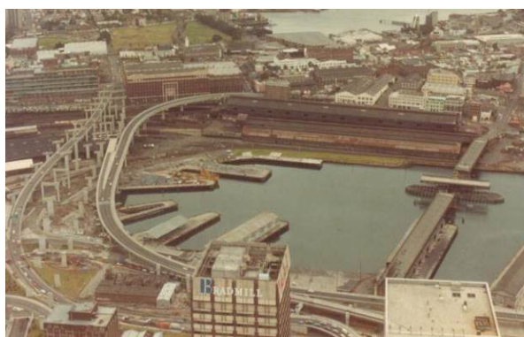
Figure 29: 1984 aerial photograph showing early stages of demolition of railway yards and wharves. 36
