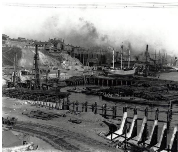
Figure 37: Example of Monier trestle seawall being constructed, Darling Harbour, 1909. 41
