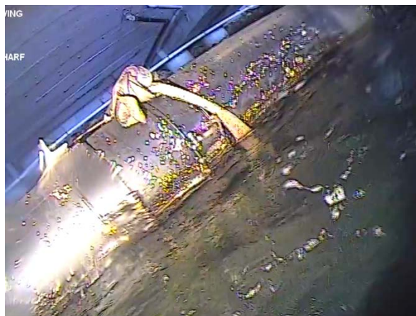
Figure 54: The rubbish net is attached to a floating drainage pipe. (Image from T1 (a) Cockle Bay 210705; 05:38).
