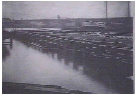
Figure 21: Wharf 35 under construction, September 1918. 28
