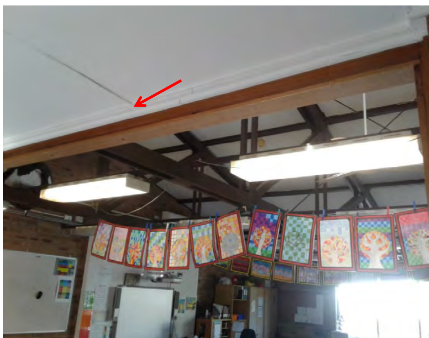
Photograph 29: B00B - R1014, Interior, Ceiling structure, White Flaking Paint, non-lead paint ( \leq 0.1\% lead w/w).
