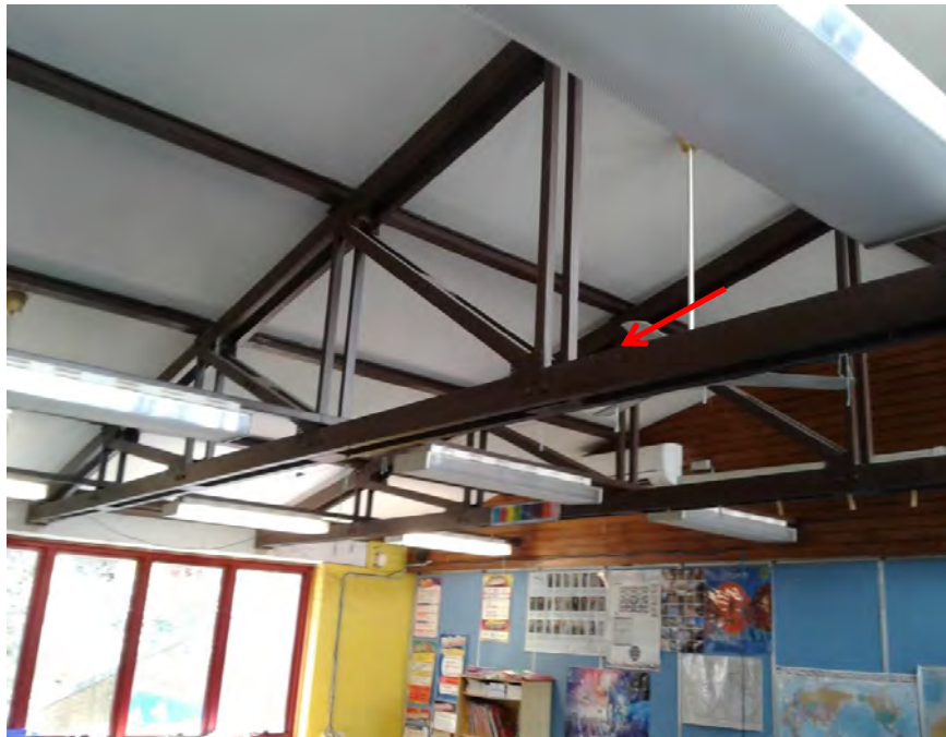
Photograph 27: B00B - R1008, Interior, Timber rafters, Brown paint, non-lead paint ( \leq 0.1\% lead w/w).
