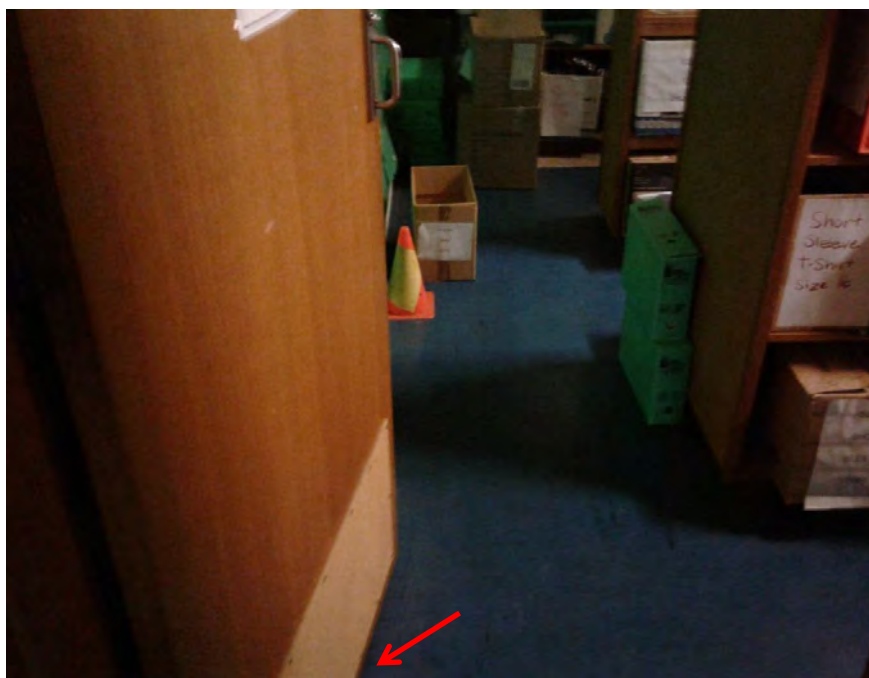
Photograph 13: B00A - R0032, Interior, Flooring material, Vinyl tiles under flooring, asbestos detected by analysis.
