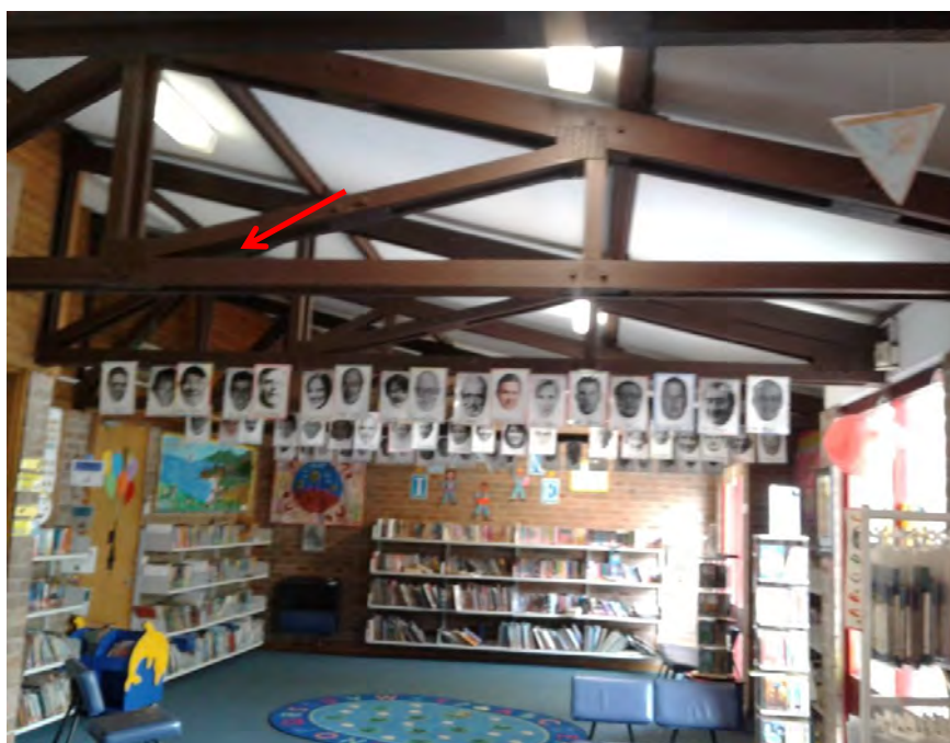
Photograph 16: B00A - R1003, Interior, Timber rafters, Brown paint, non-lead paint ( \leq 0.1\% lead w/w).
