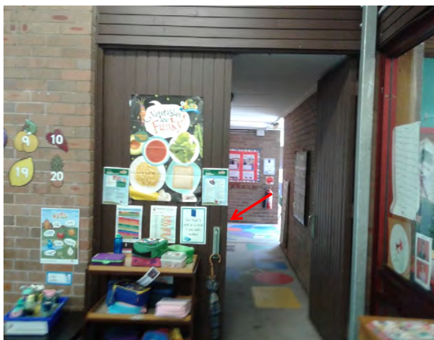
Photograph 39: B00C - R0034, Interior, Timber door, Brown Paint, non-lead paint ( \leq 0.1\% lead w/w).
