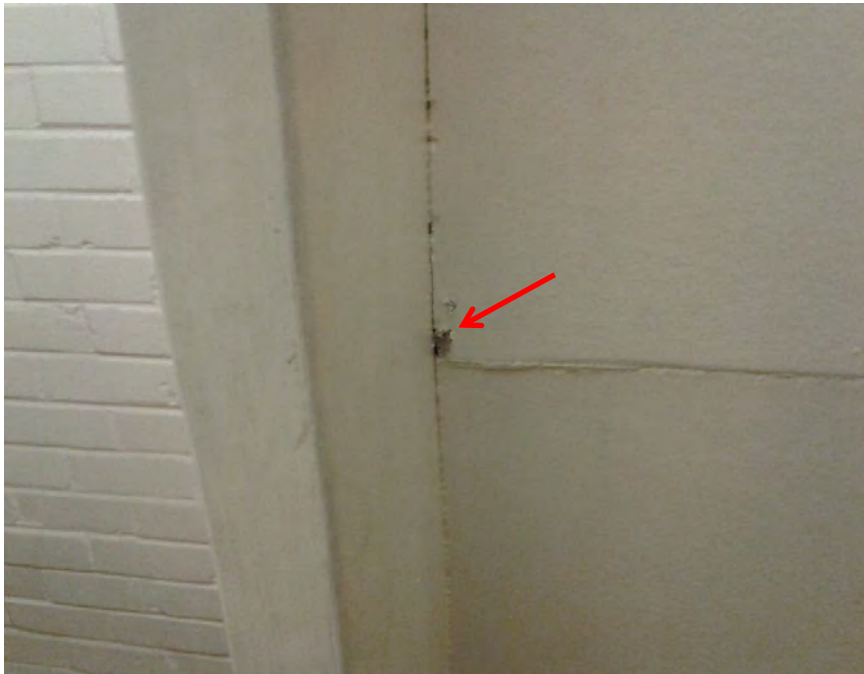
Photograph 10: B00A - R0022, Interior, Partitions in toilet, Compressed FCS sheeting, asbestos detected by analysis.
