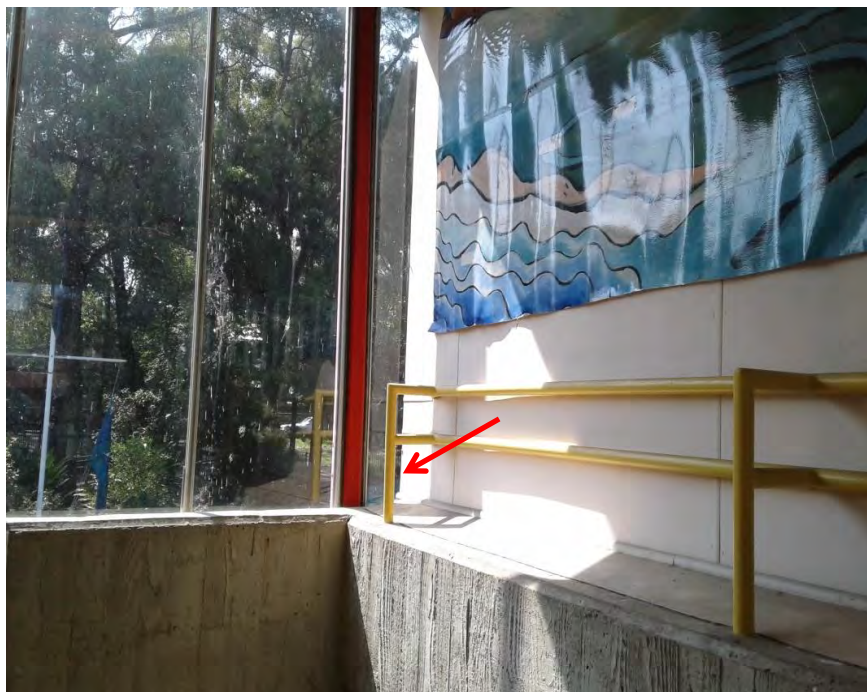
Photograph 21: B00B - R0025, Interior, FCS sheeting on wall, FCS sheeting, no asbestos detected by analysis.
