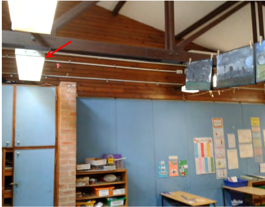
Photograph 26: B00B - R1003, Interior, Light fitting, Dust above light fitting, elevated lead ( >0.5 \text{ mg/m}^2 ).
