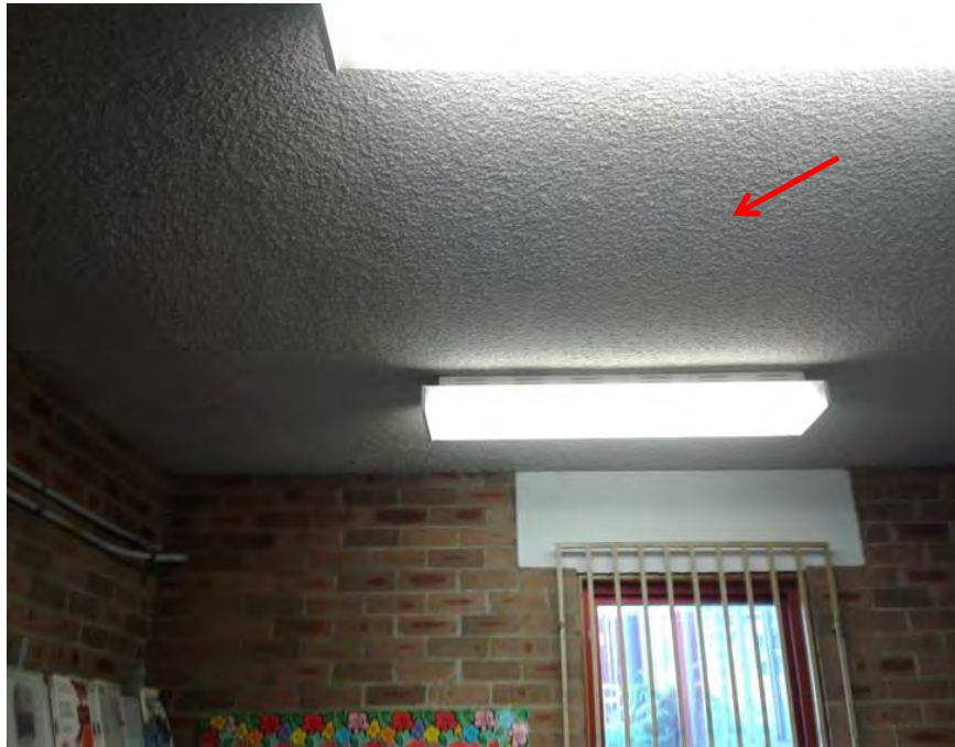
Photograph 6: B00A - R0017, Interior, Ceiling structure, Vermiculite, no asbestos detected by analysis.
