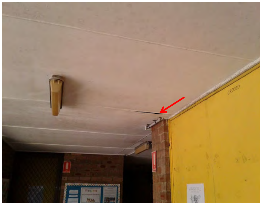
Photograph 32: B00C - R0005, Interior, Ceiling structure, FCS sheeting, no asbestos detected by analysis.
