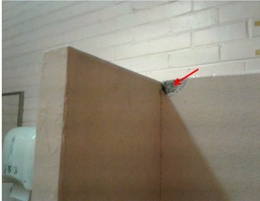
Photograph 19: B00A - R1019, Interior, Partitions in toilet, Compressed FCS sheeting, asbestos detected by analysis.
