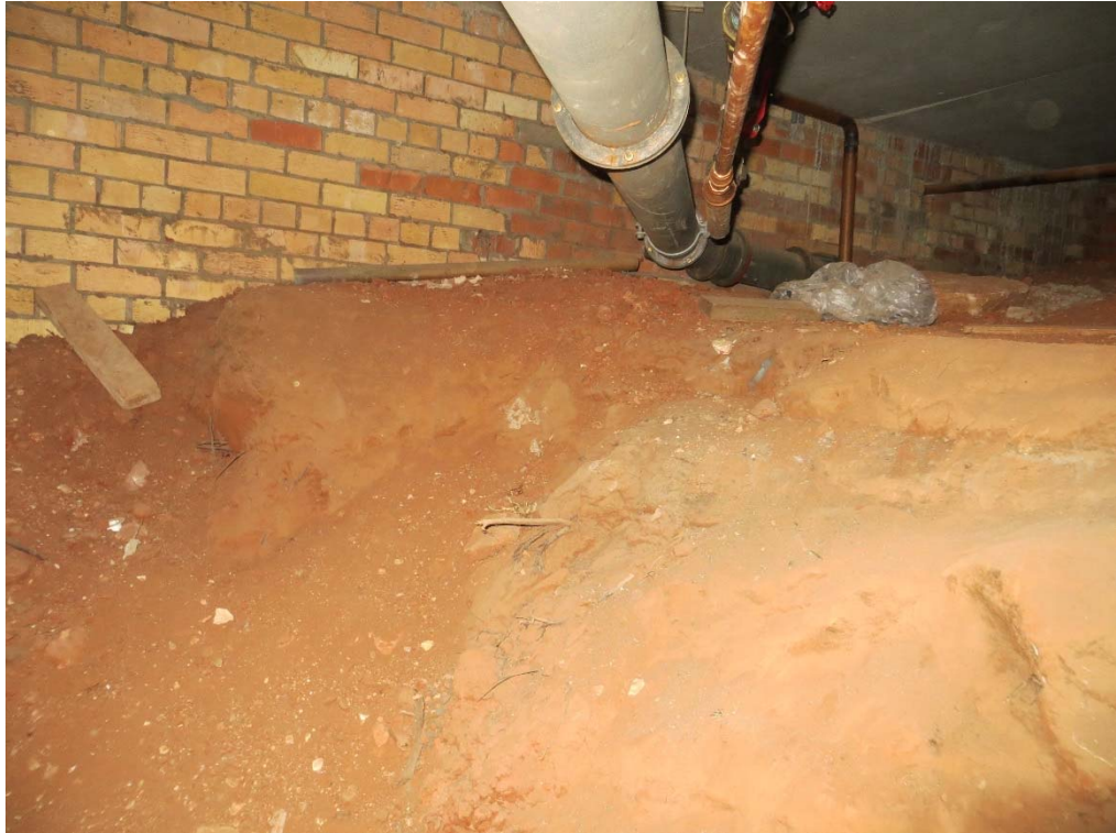
Photo 18. View of unexcavated materials or backfilled materials in the basement against the subject building wall
