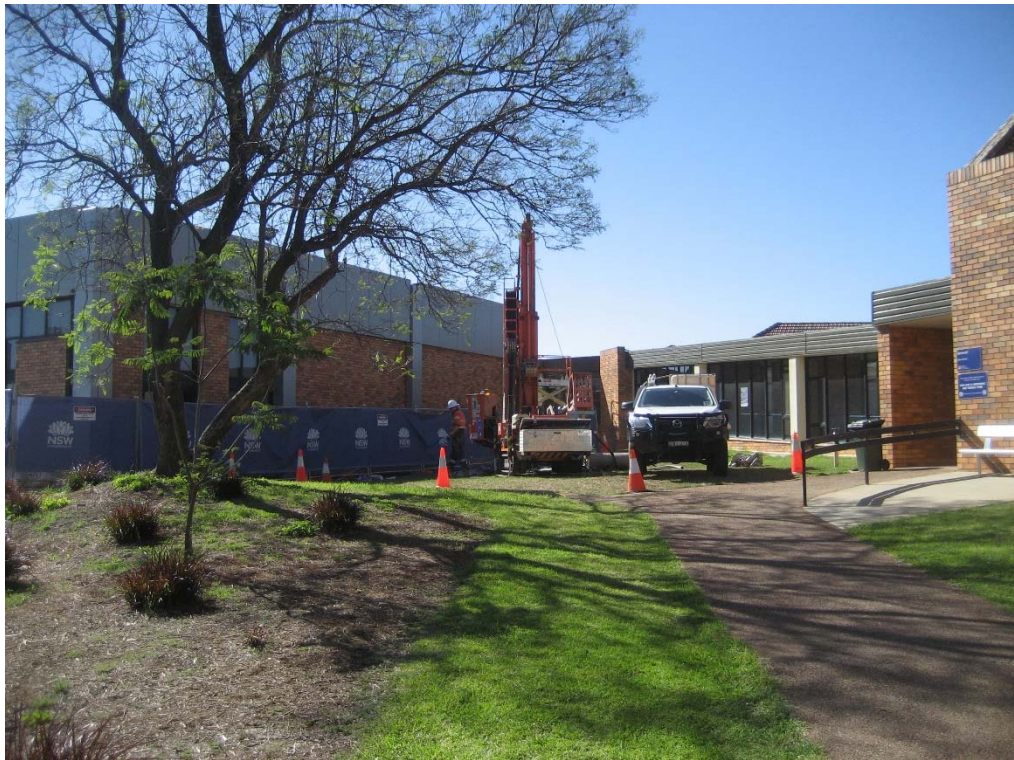
Photo 1. Drilling of BH107 in vicinity of Emergency Building
