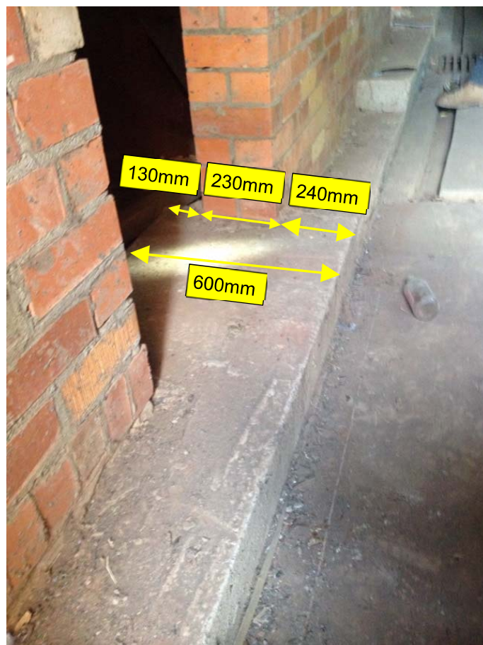
Photo 17. View of existing footing of General and Medical Ward Building
