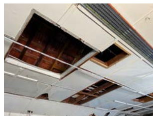
Asbestos ceiling + termite damage
