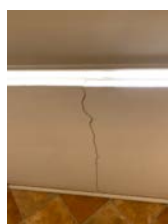
Cracked sill
