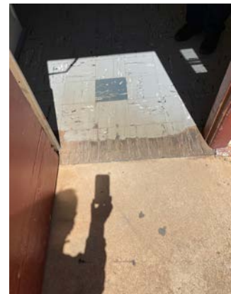
Timber overlayed vinyl tiles
