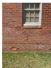
Slumped bricks (failed DPC?)
