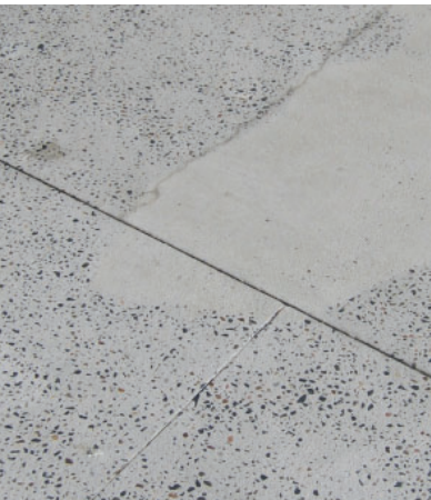
35 Exposed aggregate concrete
