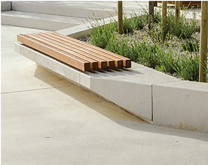
29 Precast concrete wall with timber batten seat
