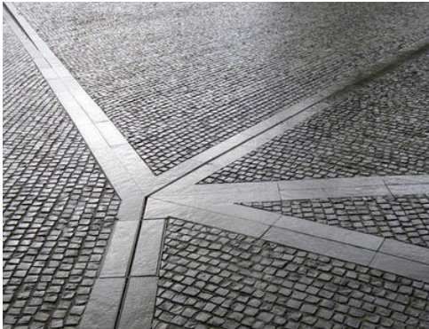
46 Zig-zag trench referenced in the paving
