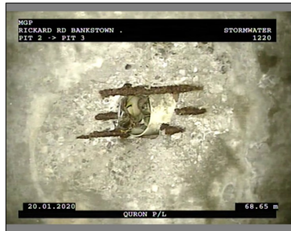
Figure 6-4 CCTV Photo Exposed Reinforcement
