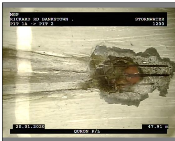
Figure 6-1 CCTV Photo Exposed Reinforcement
