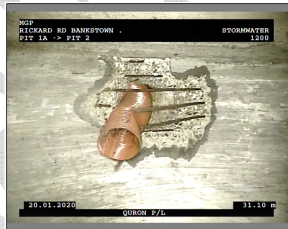
Figure 6-2 CCTV Photo Poor Connection Workmanship
