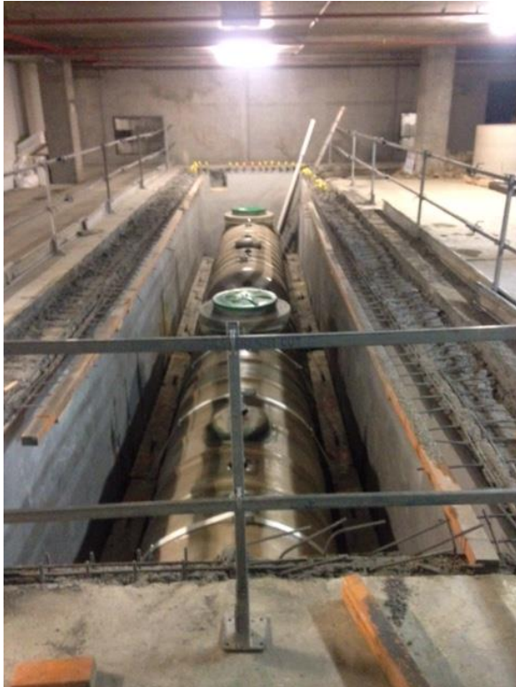
Figure 3. Underground chamber for diesel tanks showing the steel straps and concrete anchors.
