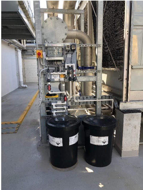
Figure 11. Chemicals connected to dosing equipment.
