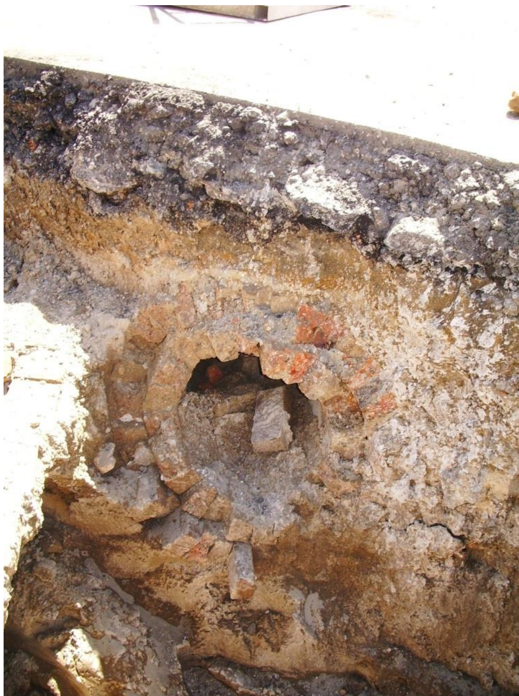
Figure 3.5 Circular brick drain exposed during roadworks in 2012, in the roadway at the southwest corner of the intersection of Church and Newcomen Streets. AMAC, 2012, digital 0991.
