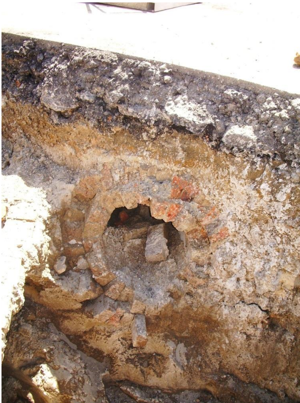
Figure 3.12 Circular brick drain exposed during roadworks in 2012, in the roadway at the southwest corner of the intersection of Church and Newcomen Streets. AMAC, 2012, digital 0991.
