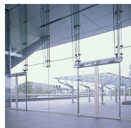
02. Tempered Glass, Glass Rib Structure
