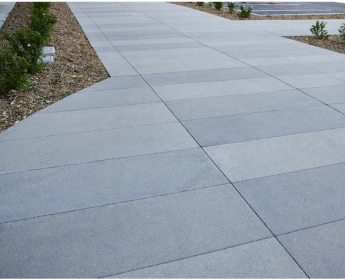
Concrete paving with saw cut
