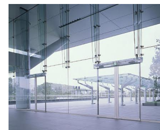
04. Tempered Glass, Glass Rib Structure
