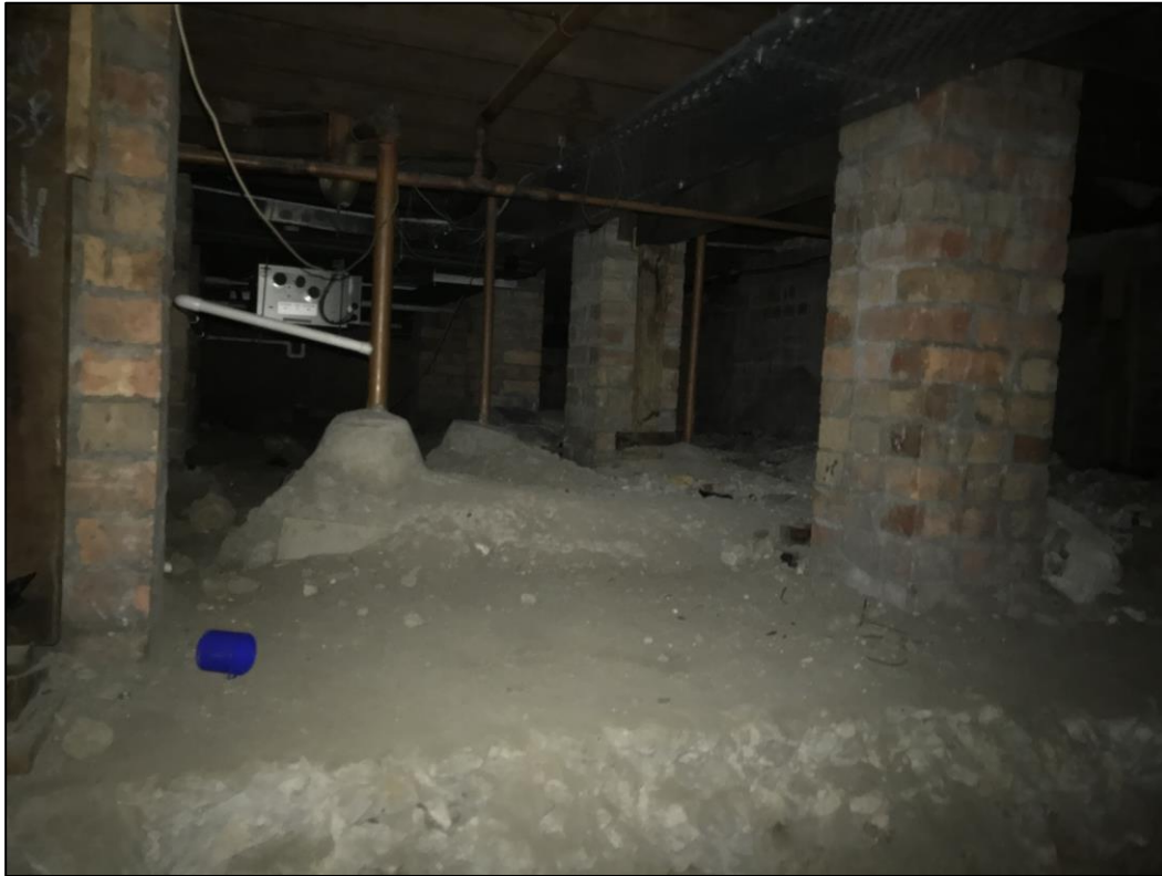
Figure 5.3 Basement level indicating depth of footings and services. No intact soil evident. AMAC (2019) IMG_8956
