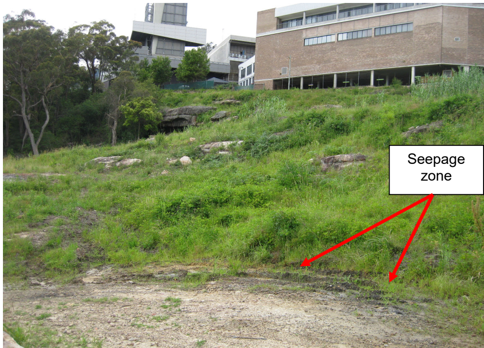
Photo 9 – View south-east from the winding access track, towards a zone of seepage onto the access track as indicated.
