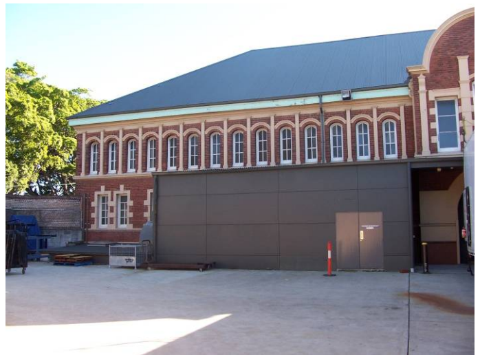
Figure 23 View of the south façade showing the 1990s enclosure of the external staircase to the basement toilets.
