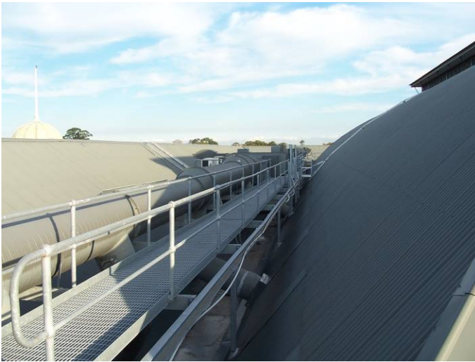
Figure 20 View looking south along eastern roof valley showing elevated access walkway, air handling equipment and ductwork.
