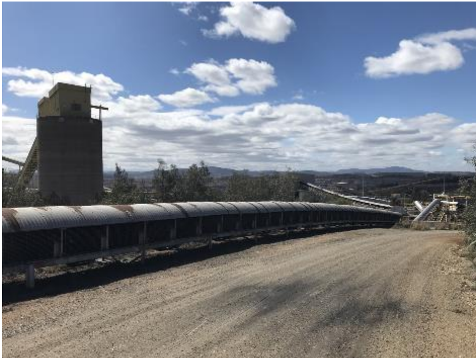
Figure 5-1: Vehicle track and working coal conveyor (ash line out of frame to right) (Source: Jacobs 2019)
