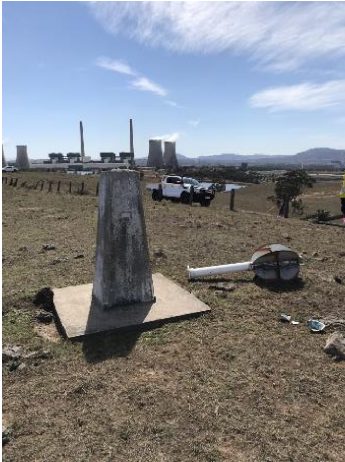
Figure 5-9: Derelict trig station (mast and vanes broken off and lying on the ground; Bayswater at rear of frame), looking north (Source: Jacobs 2019)
