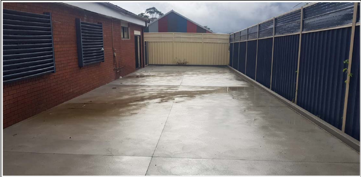
Figure 3 | Completed hardstand capping layer (Source: submitted SVR prepared by Agility Engineering)
