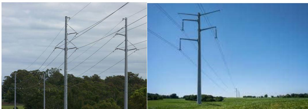
**Figure 3-11 Typical Steel Pole Structures, Transmission Line**
