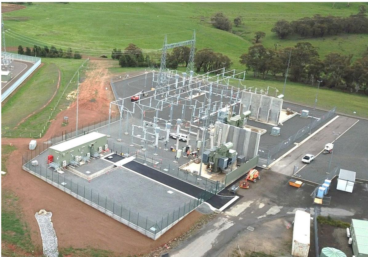
**Figure 3-12 Typical Substation - Gullen Range Wind Farm 33/330kV Substation**
