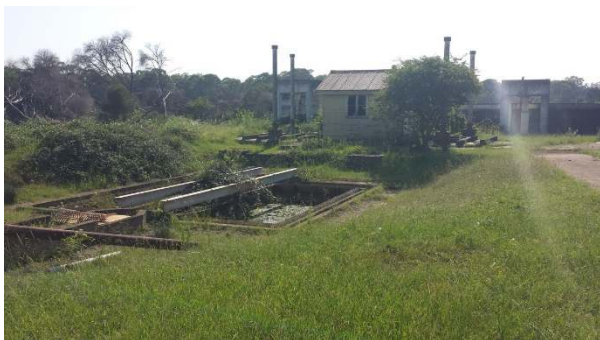
Figure 31. Sewage treatment plant: sedimentation tanks
