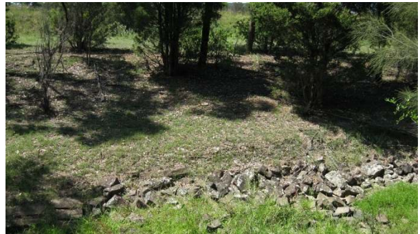
Figure 26. Rock infill to prevent erosion
