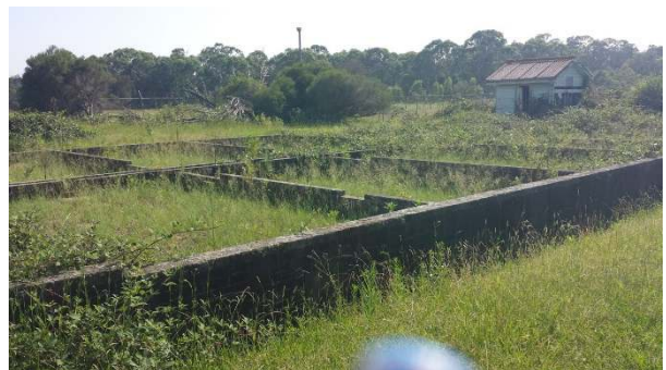
Figure 32. Sewage treatment plant: Sludge drying tanks
