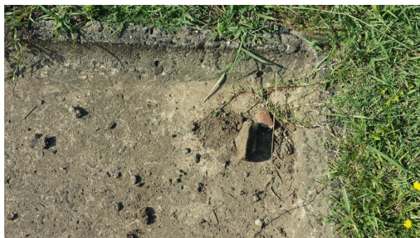
Figure 42. Detail of slab showing bluestone concrete, curved lip and isolated artefact (ink bottle sherd)
