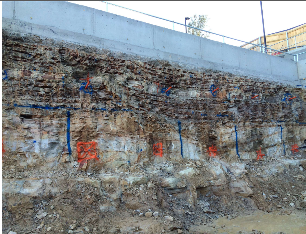
Photo 1: Excavation face in highly weathered Mittagong Formation and Hawkesbury Sandstone
