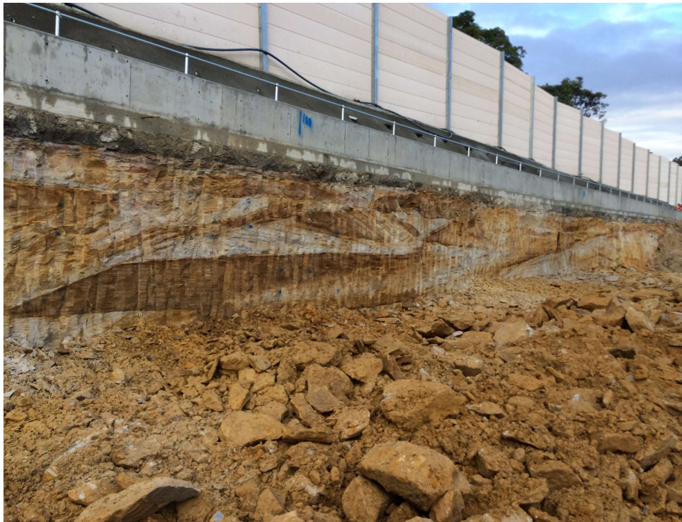
Photo 2: Vertical excavation face in moderately weathered Hawkesbury Sandstone
