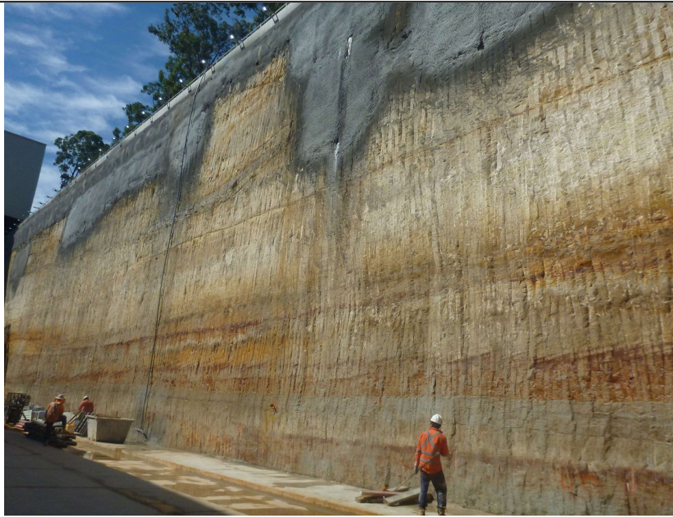
Photo 3: Vertical excavation face in fresh Hawkesbury Sandstone excavated by rock hammer
