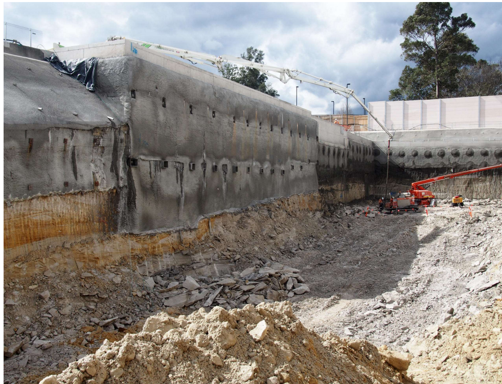
Photo 4: Typical excavation support in sandstone (cut batter, pattern rockbolts, shoring piles with anchors)
