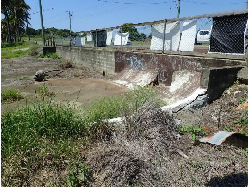
Plate 5. Concrete slab and block retaining wall along Cudgen Road boundary, looking east.
