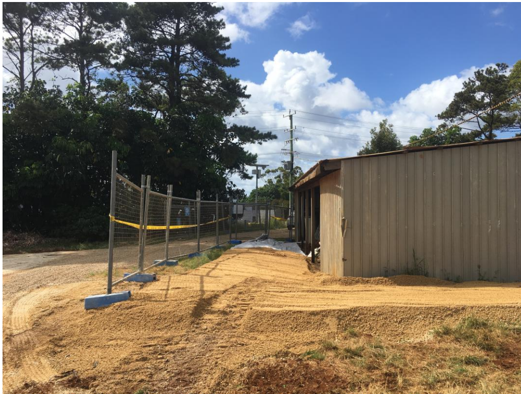
Photograph 3. View east of geofabric and gravel placed around the farm shed.
