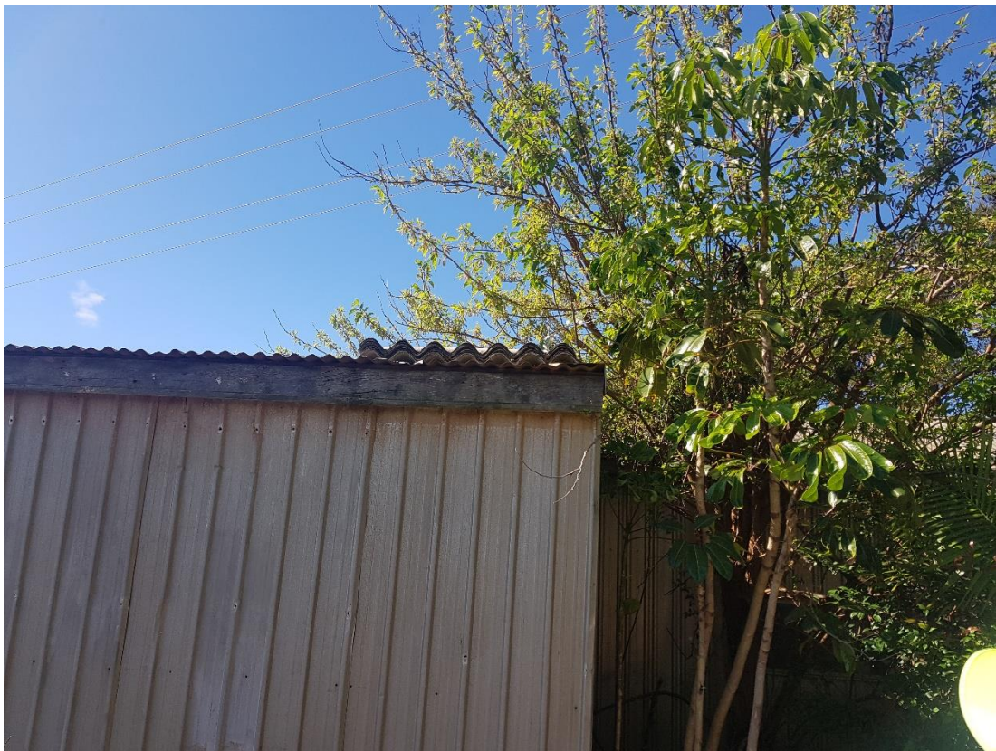
Photo 2 – Asbestos containing sheeting on roof of storage shed building.
