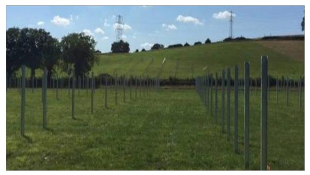
Figure 4-3: Piles for the solar farm in place (image source Infinergy UK)
