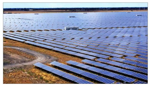
Figure 4-4: Fully assembled tracking array solar farm showing inverter housing (image courtesy Nextracker Australia, actual tracking system may differ)
