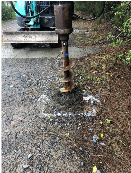
Photo 1: Placement of Borehole using 300mm Auger Attachment
