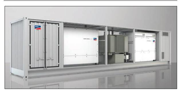
Figure 3-11 Containerised inverter/transformer unit with battery storage (SMA)
