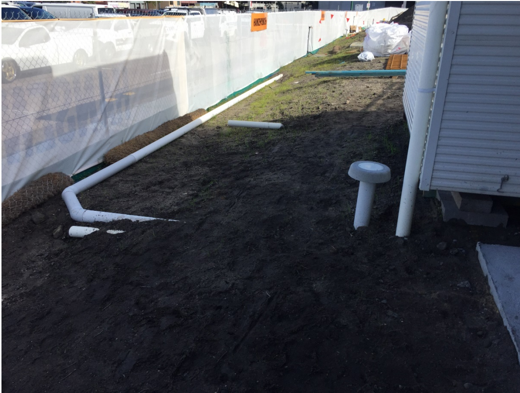
Photo 15: Sediment and erosion controls along site boundary (southern fence)
