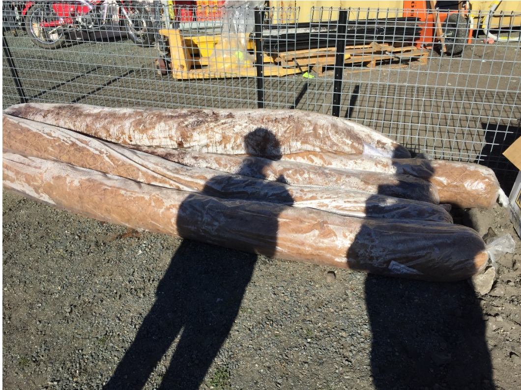
Photo 12: Spare sediment and erosion controls (booms)
