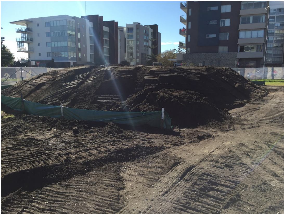
Photo 8: Stockpile area with sediment fence control
