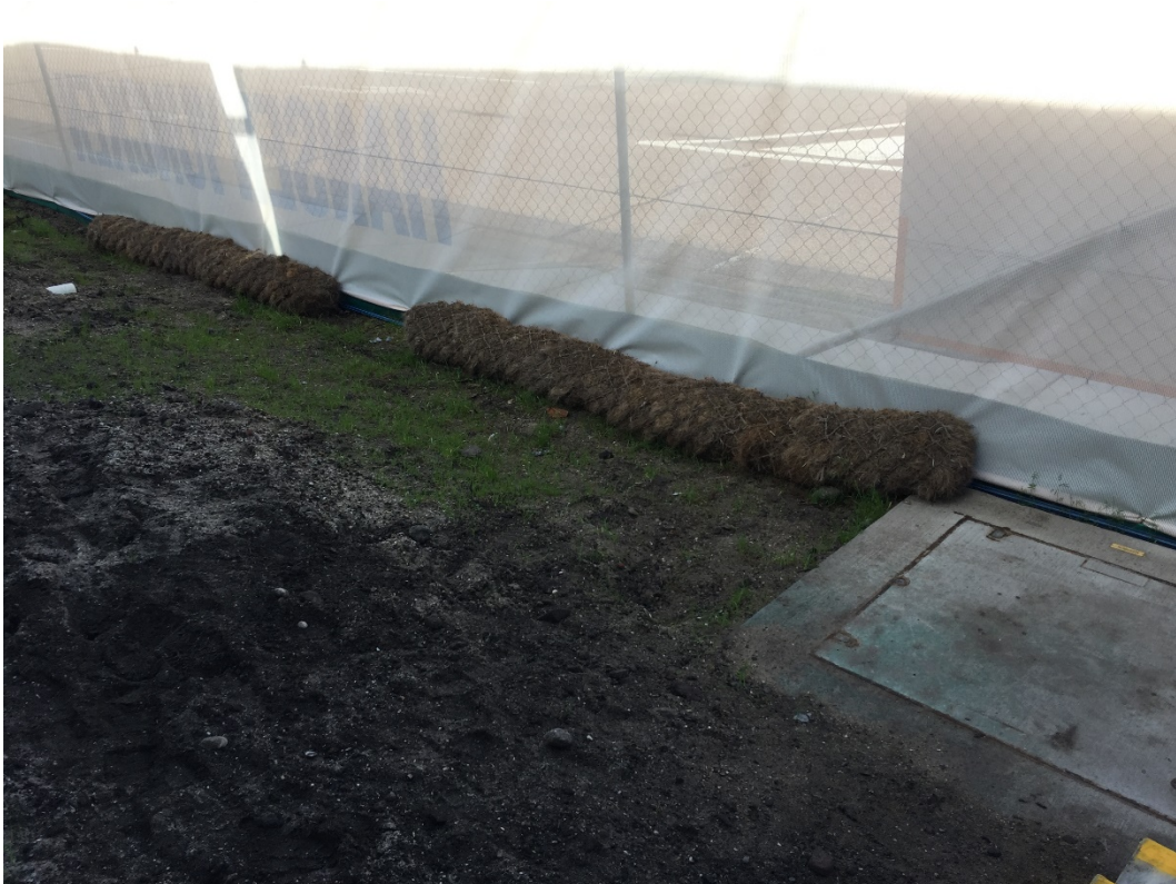
Photo 14: Sediment and erosion controls along site boundary (southern fence)
