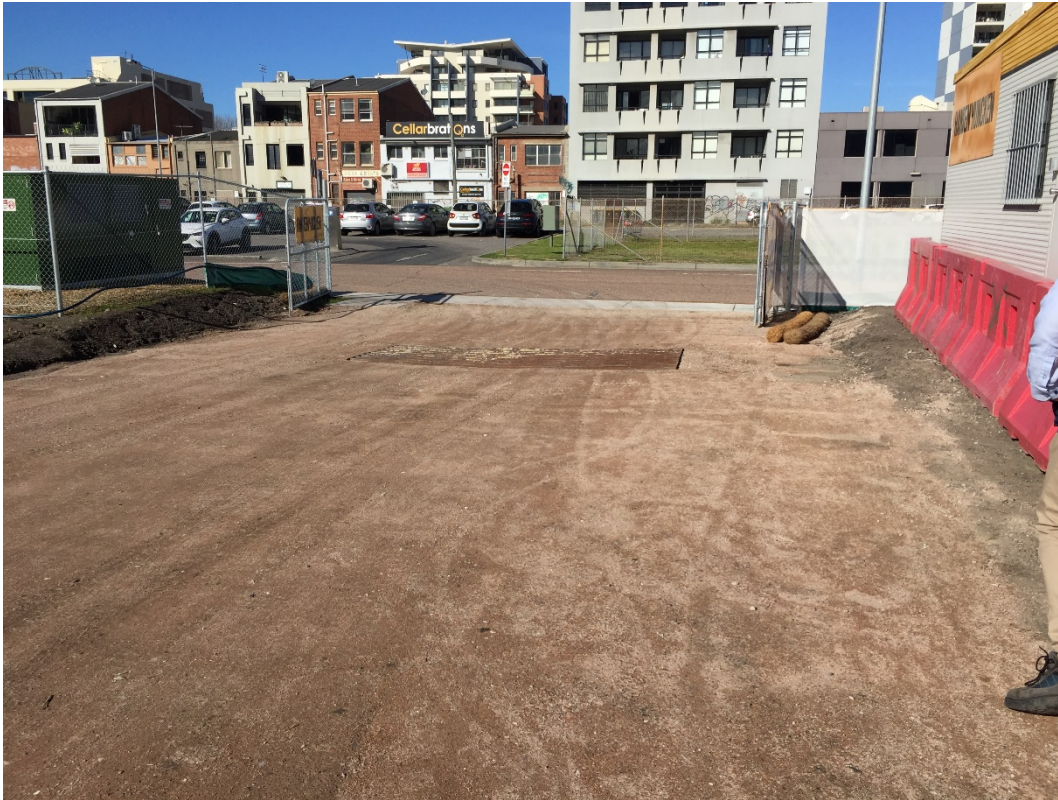
Photo 13: Cattle grid at site vehicle entry/exit
