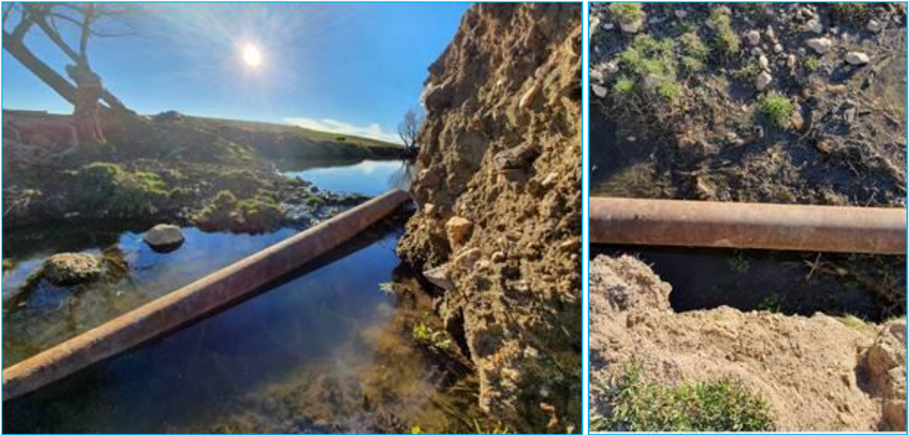
Plate 4.4 Evidence of existing impediment to fish passage (55H 713524 6292895) upstream of BR-07, Belubula River
