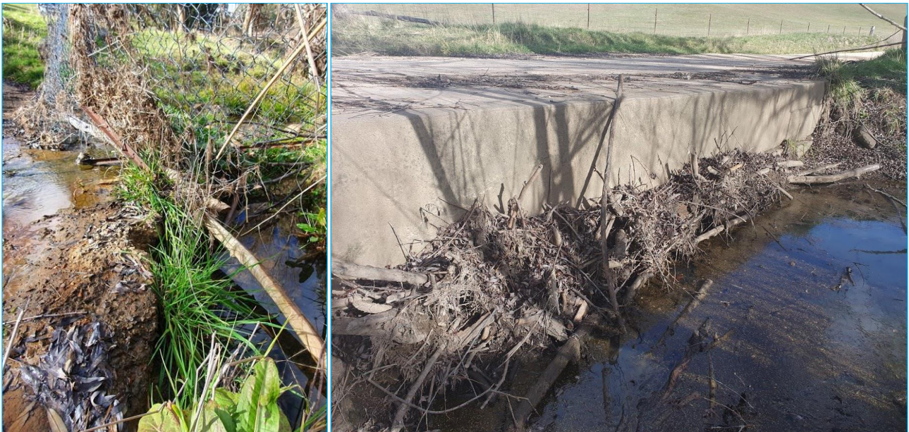
Plate 4.1 Evidence of existing impediment to fish passage (Dungeon Road causeway) upstream of BR-04, Belubula River
