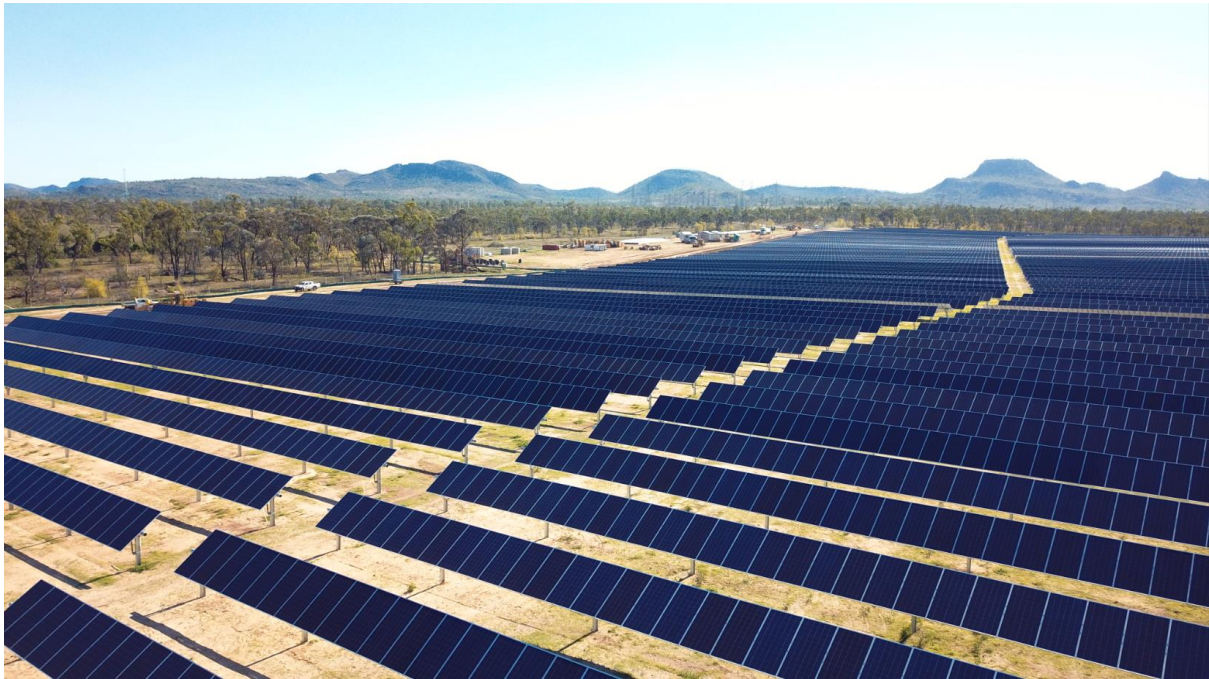
Figure 5: Example of a single axis tracking system (Wirsol owned Hamilton Solar Farm in QLD)
