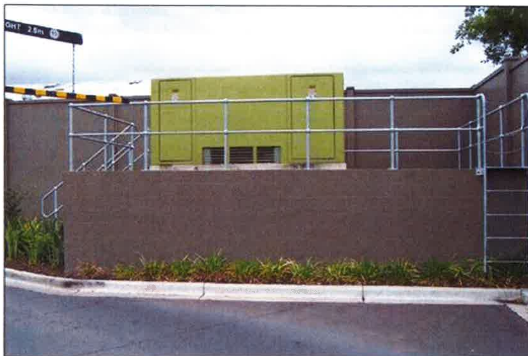
Figure 51 - Example substation raised above 1:100 flood level
