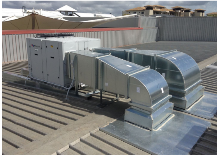
Figure 7: Example of rooftop packaged air-conditioning system
