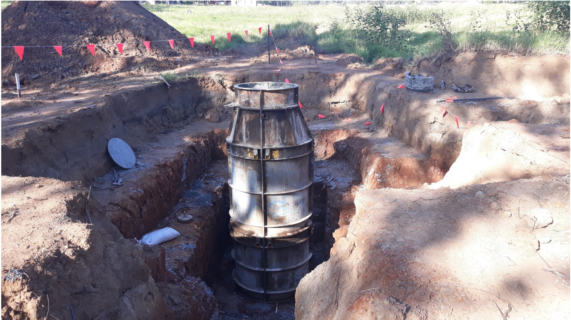
Figure 8-3 Sewage cistern installed below dam on proposal site
