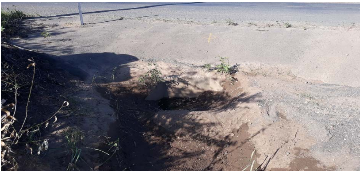
Figure 4-4 Degraded culvert clogged with sediment
