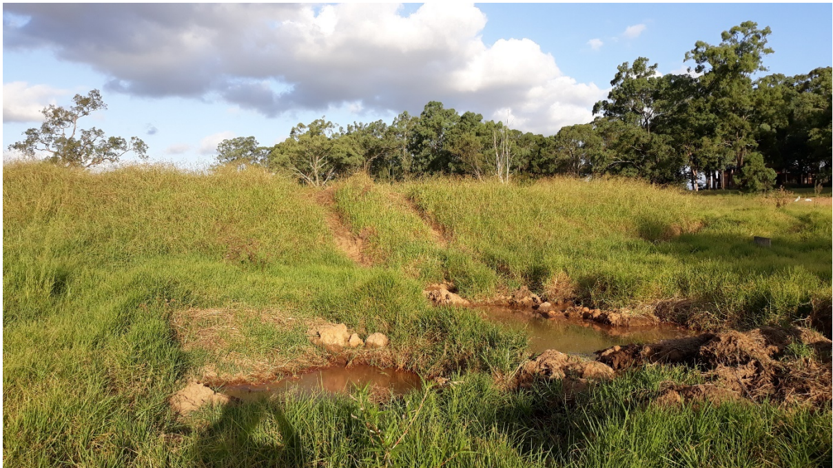
Figure 4-10 Water seepage in ground disturbance below the dam wall
